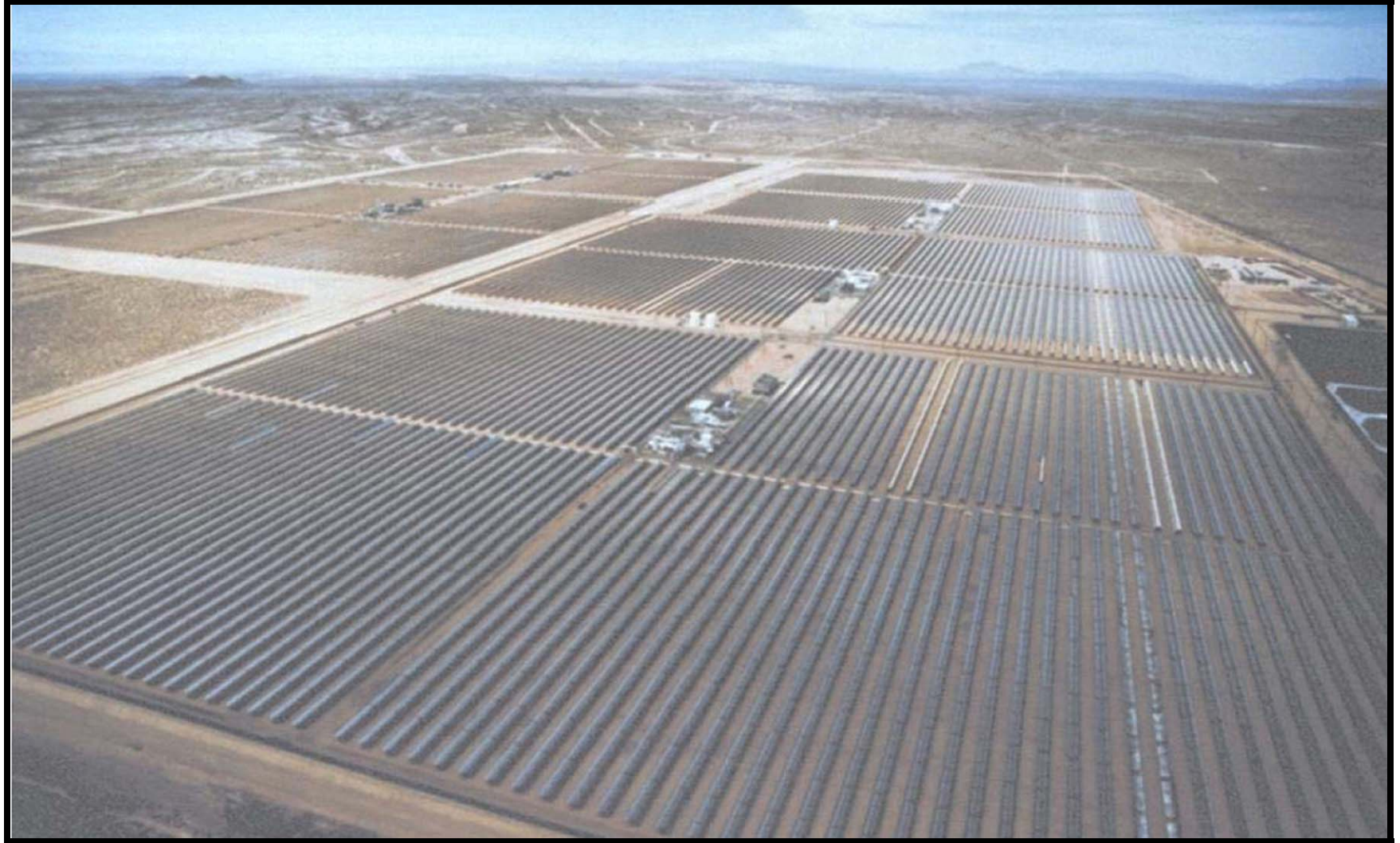
Figure 7: Picture of Similar Solar Generating Facility (Kramer Junction Solar Plant)
