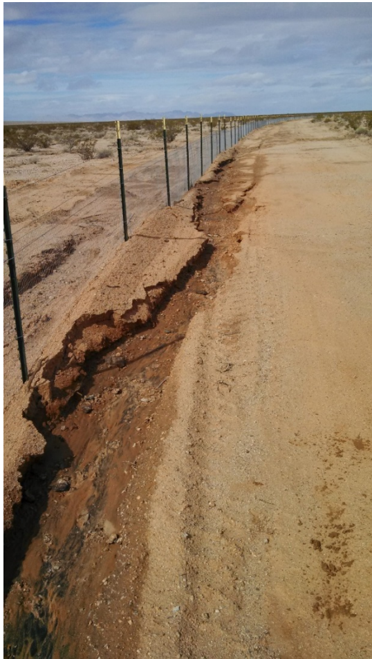
LOCATION 2. UTM 701777 E, 3770406 N, DATUM WGS 83 VIEW WEST
