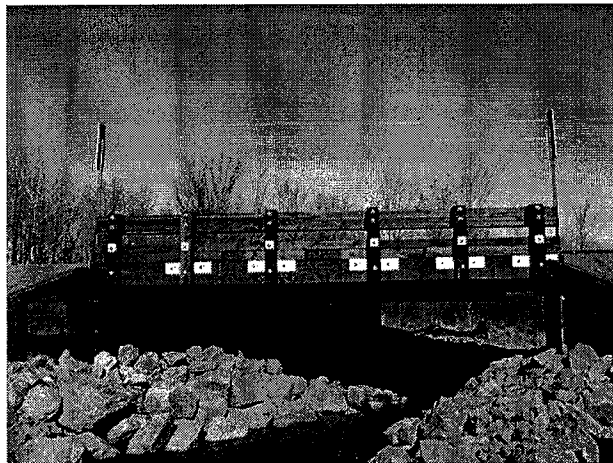
Overall Elevation New FHWA/AASHTO Approved Timber Trestle Bridge in Wisconsin
