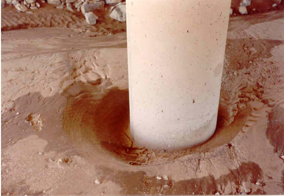
Figure 5. Local scour around bridge pier
