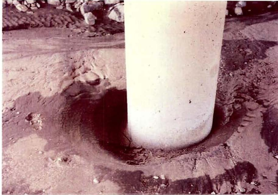
Figure 9. Local scour around bridge pier
