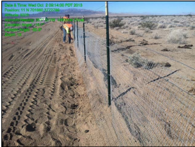
Figure 2a and 2b- Desert Tortoise Fence Modification
