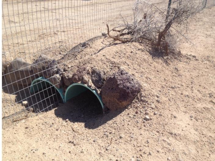
**Figure 2: Desert Tortoise Shade Structure Installed along Rice Solar Energy Project Perimeter Fence**
