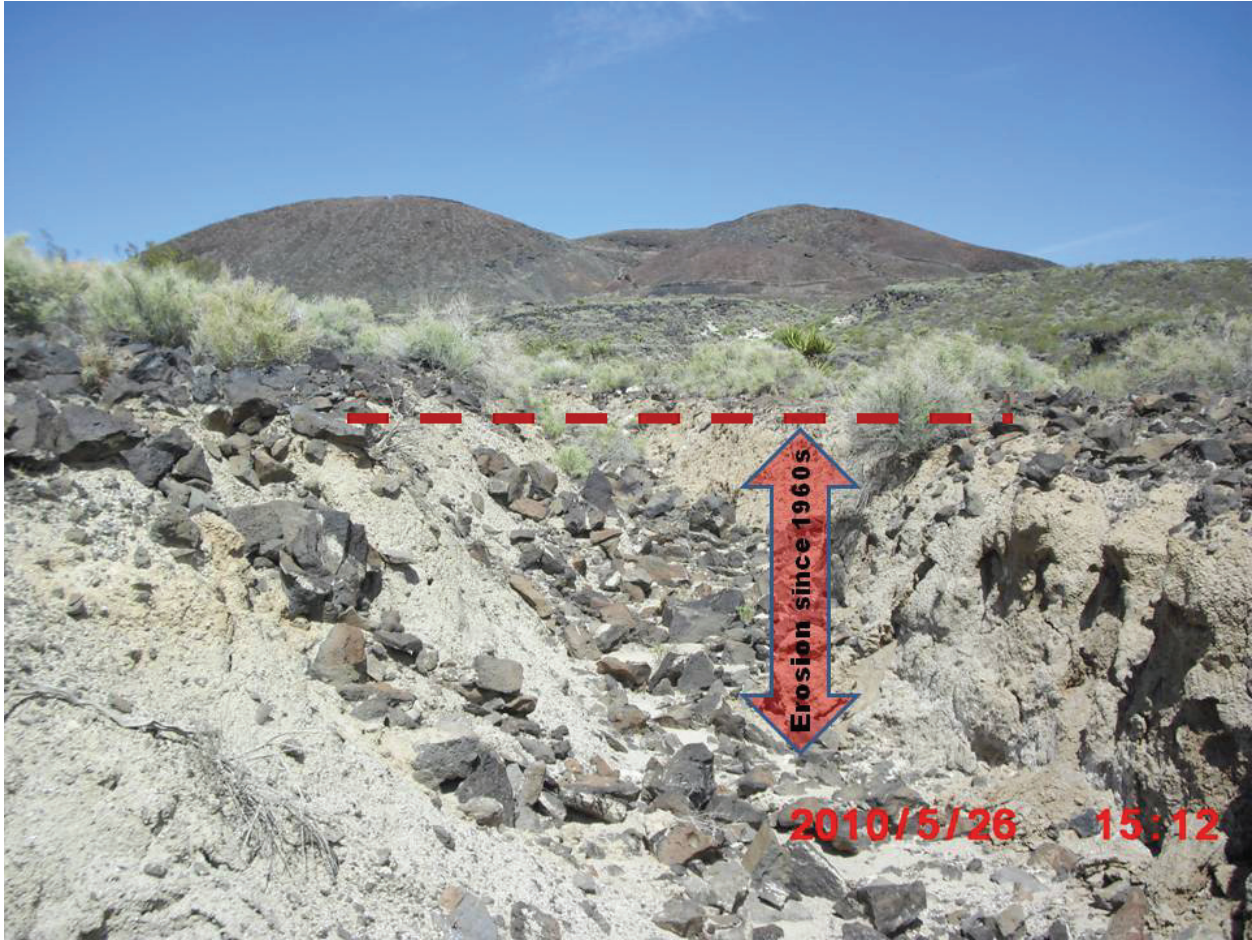
Figure 1: Erosion caused by run-off along a mining road where desert pavement was removed in the 1960s. Here the top layer was simply bulldozed to the side exposing the accumulated Av Horizon. This mining road is located approx. 45 miles north-east of the project area. The pre-mining road conditions of this area were flat and uninterrupted.
