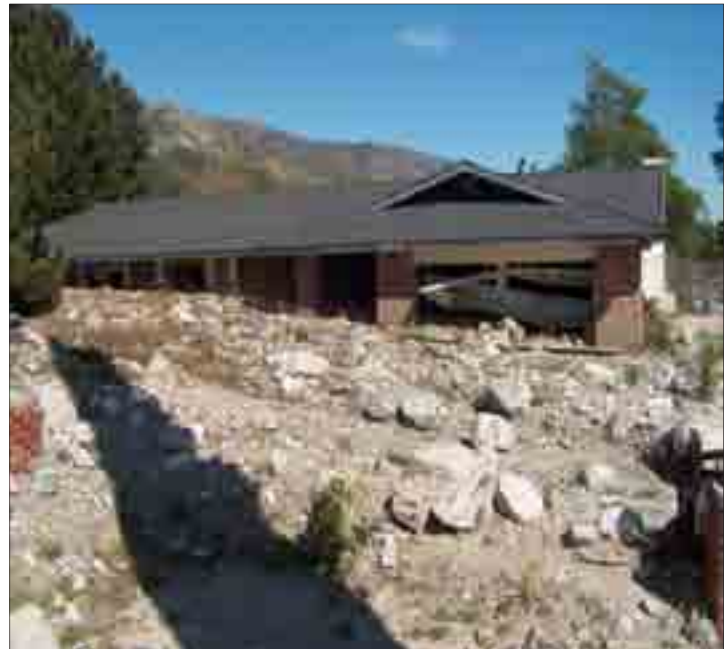
Figure 4: A house in San Bernardino County is inundated by a debris flow following a heavy rain event on Christmas Day after the 2003 wildfires. Source: Dr. Norman Meek, California State University, San Bernardino
