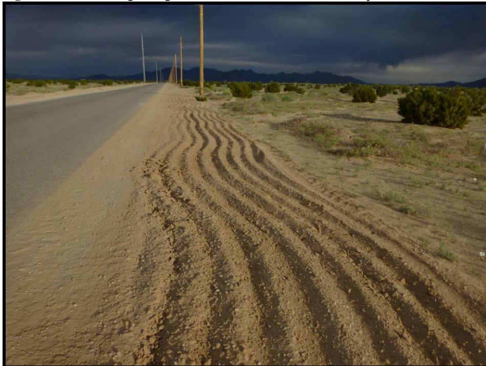
Figure 2c. Surface roughening to create sediment and moisture traps.
