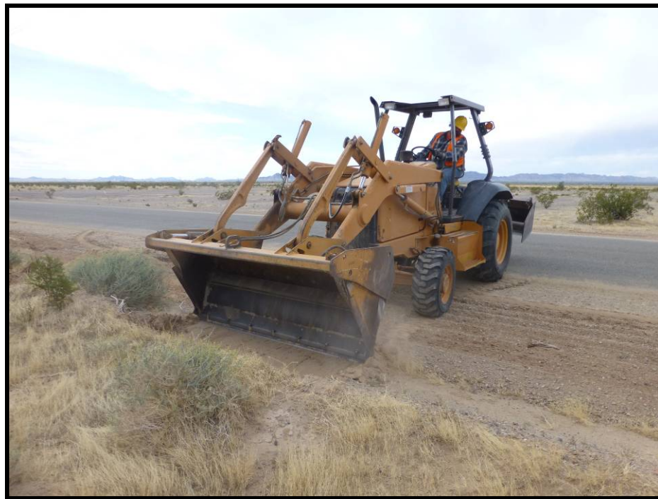
Figure 2a. The gannon spreading the topsoil berm over the ripped, decompacted shoulder
