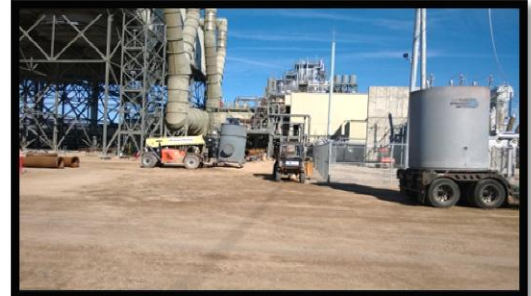
Power Block 1 – Steam Blow Piping
