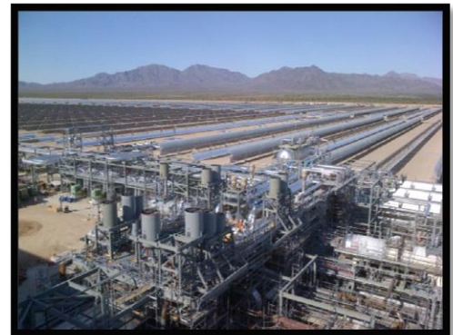
Power Block 1 – Area 23
