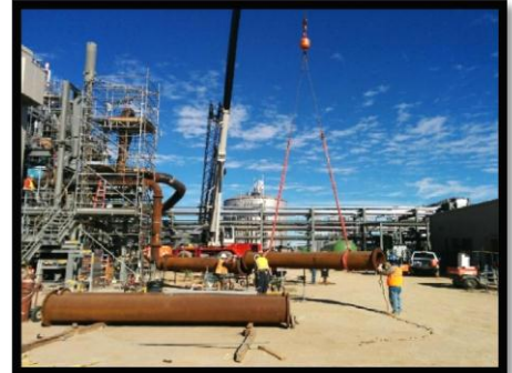
Power Block 1 – Steam Blow Pipe Install
