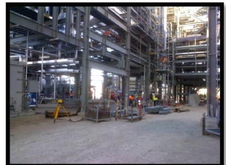
Power Block 1 – Area 26
