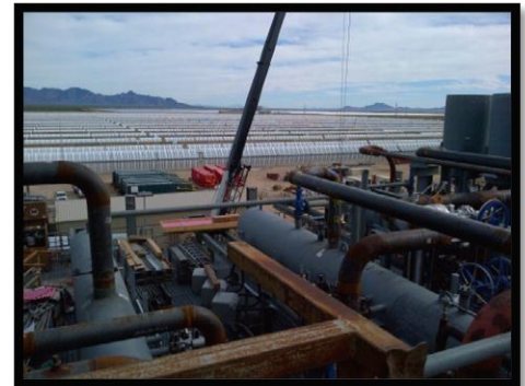
Power Block 1– Feed Water Structure
