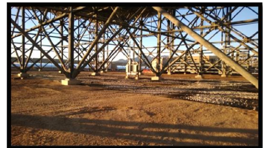
Power Block 1 – ACC Rock
