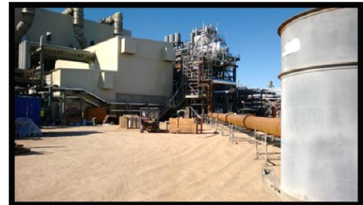
Power Block 1 – Area 11
