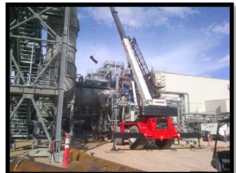
Power Block 1 – Steam Blow Piping
