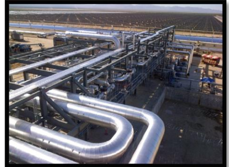
Power Block 1 – Area 22
