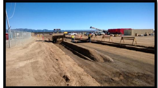
Power Block 1 – Base Installation
