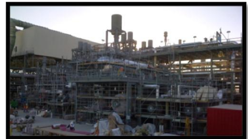
Power Block 1 – Area 15
