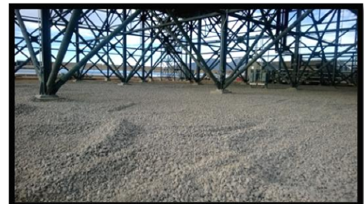
Power Block 1 – Area 20
