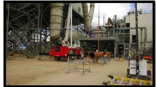
Power Block 1 – Steam Blow Piping
