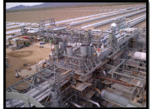
Power Block 1– Area 23
