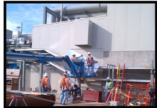
Power Block 1– Area 11
