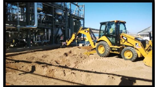
Power Block 1 – Area 16
