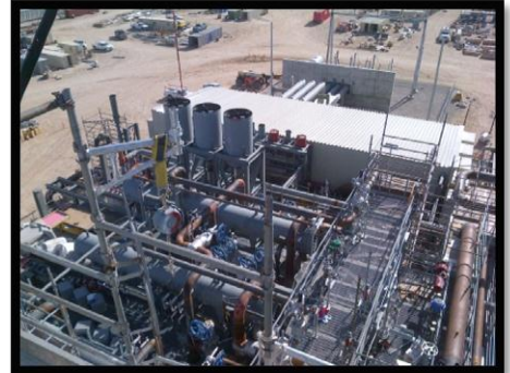
Power Block 1 – Area 14
