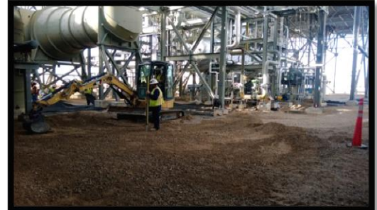
Power Block 1 – Area 26
