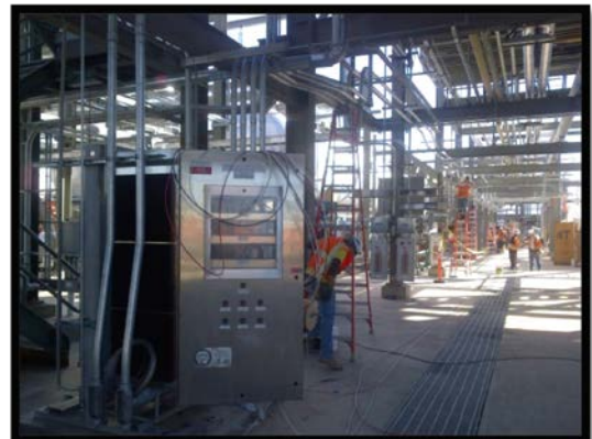
Power Block 1-Heat Trace Wire Pull
