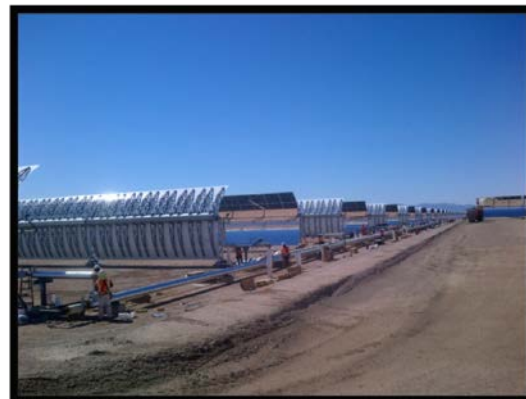
Solar Field 1 Block 6 Header Pipe Insulation
