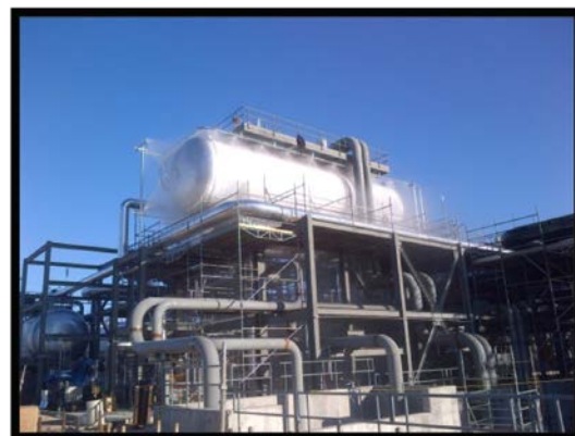
Power Block 1 Expansion Tank Spray Pattern Test
