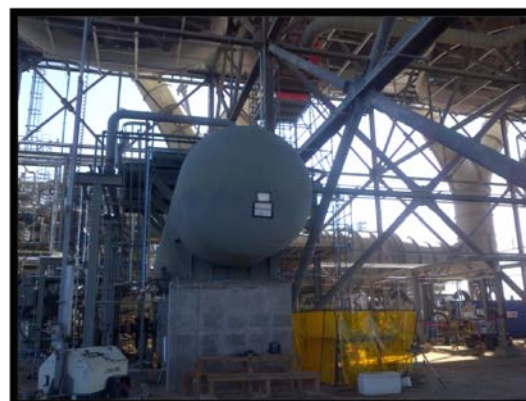
Power Block 1 ACC Condenser Tank
