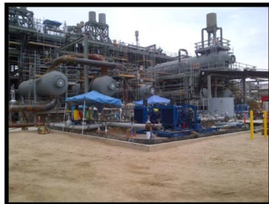
Power Block 1 Chemical Clean Equipment Set up
