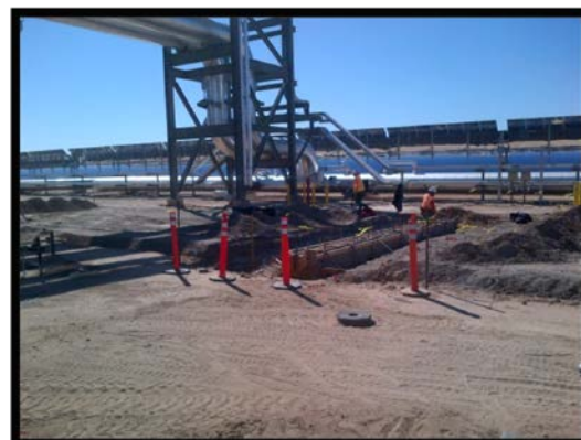
Power Block 2 Trench Drains
