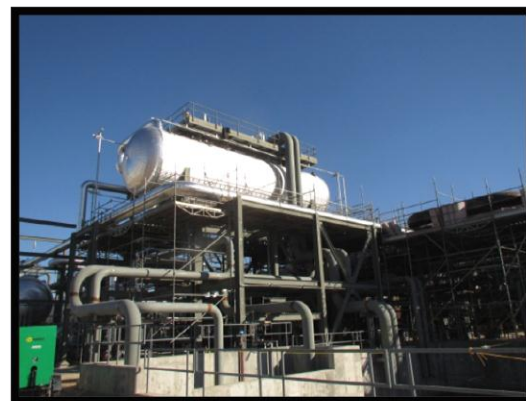
Power Block 1 – Expansion Vessel
