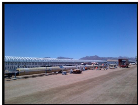
Solar Field 1 – North/South Header Insulation
