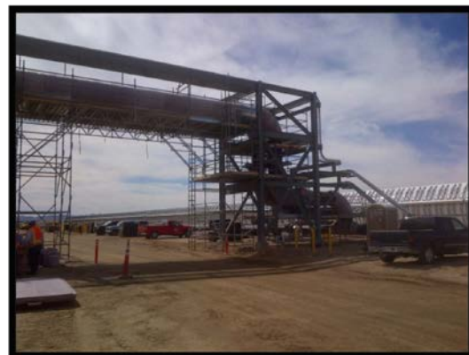
Power Block 1 Main HTF Header
