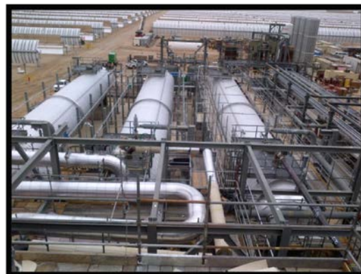
Power Block 1 HTF Overflow Vessels and Piping
