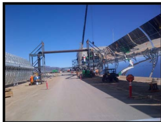
Solar Field 1-Installing pipe on Bridge 2
