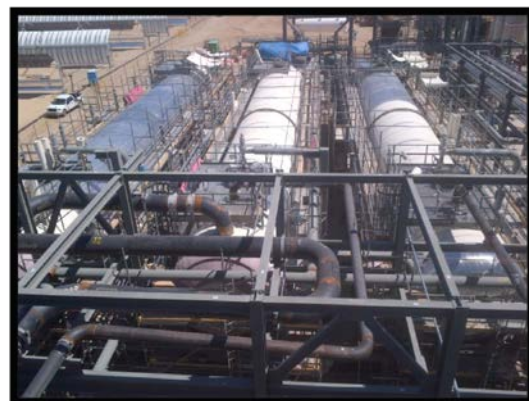
Power Block 1 Overflow Vessels
