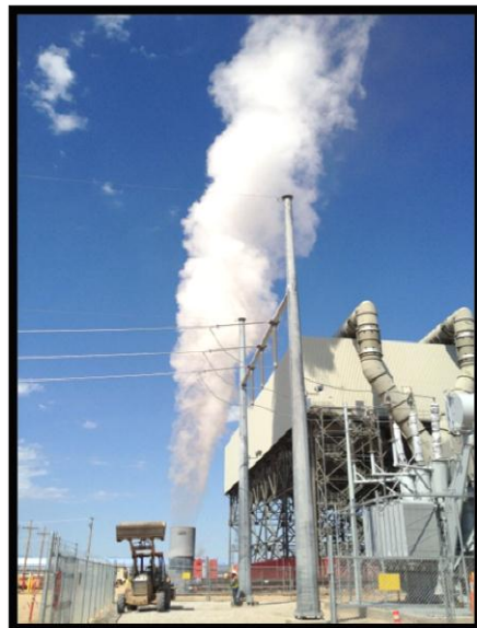
Power Block 2 Steam Blows
