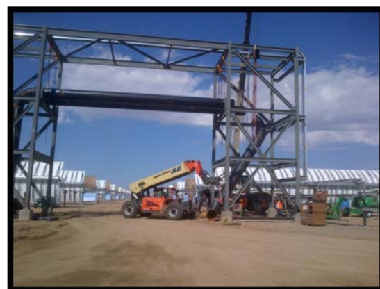
Solar Field 2- Installing Header Pipe on Bridge 3
