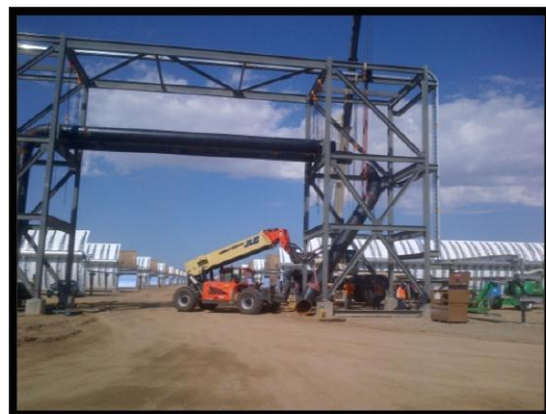
Solar Field 2- Installing Header Pipe on Bridge 3
