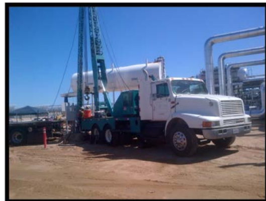
Unit 2-Permanent Well Install
