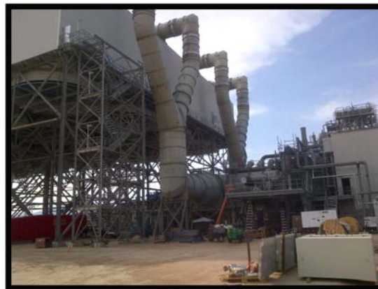
Power Block 2 Air Cooled Condenser
