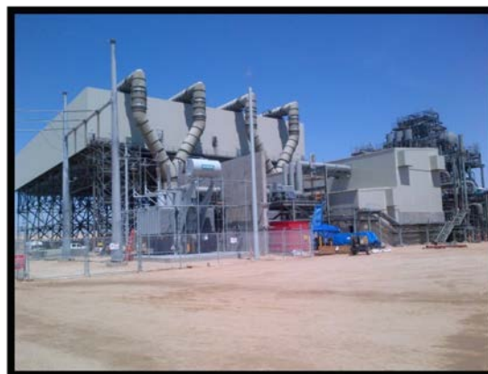
Power Block 2 Main Transformer
