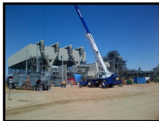
Power Block 2- Offloading Steam Blow Silencers
