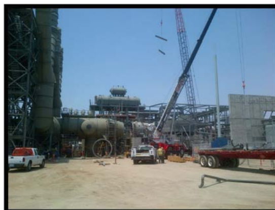
Power Block 1-Installing Steel on Boiler Feed Water Structure
