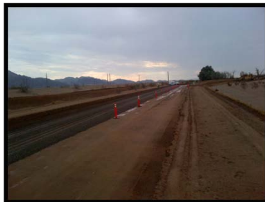
Cal Trans ROW Aggregate Base Placement
