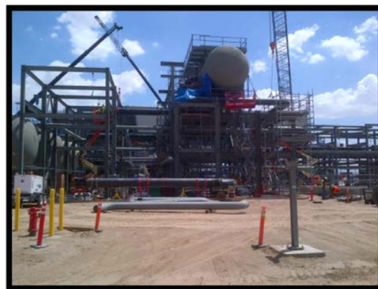
Power Block 1 Expansion Tank Piping
