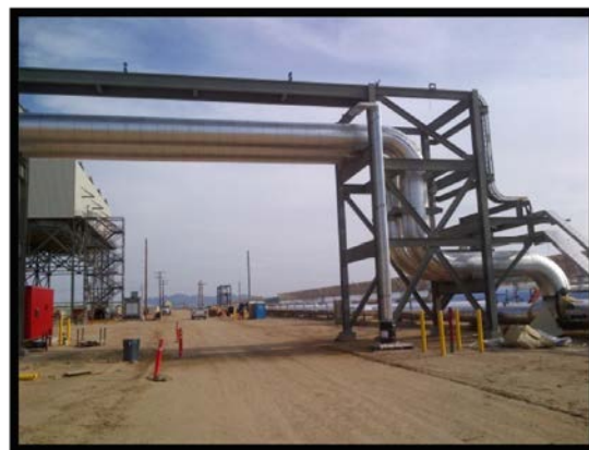
Power Block 2 and Solar Field 2 HTF Pipe Tee
