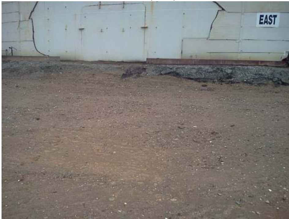
Photo 1: Location of soil pit prior to excavation.
