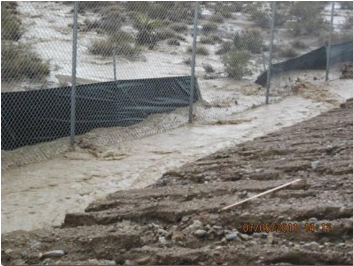
^Ivanpah Solar Electric Generating System: desert tortoise exclusion fence removed by floods. July, 2011
