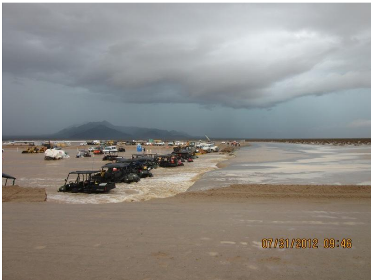
^The biggest flood took place at NextEra's Genesis Project on July 31 st , 2012. The close proximity to a dry lake and alluvial fans make this project location one of the poorest choices to site a large solar project.
