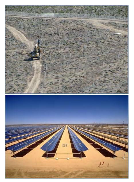
Figure DR 86-1. Minimal ground disturbance of power tower technology solar field relative to parabolic trough solar field
