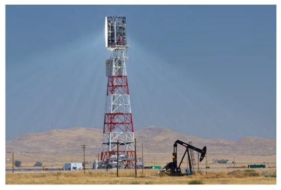
Figure DR 151-1. Visual scattering at the Coalinga Solar-to-Steam Facility
