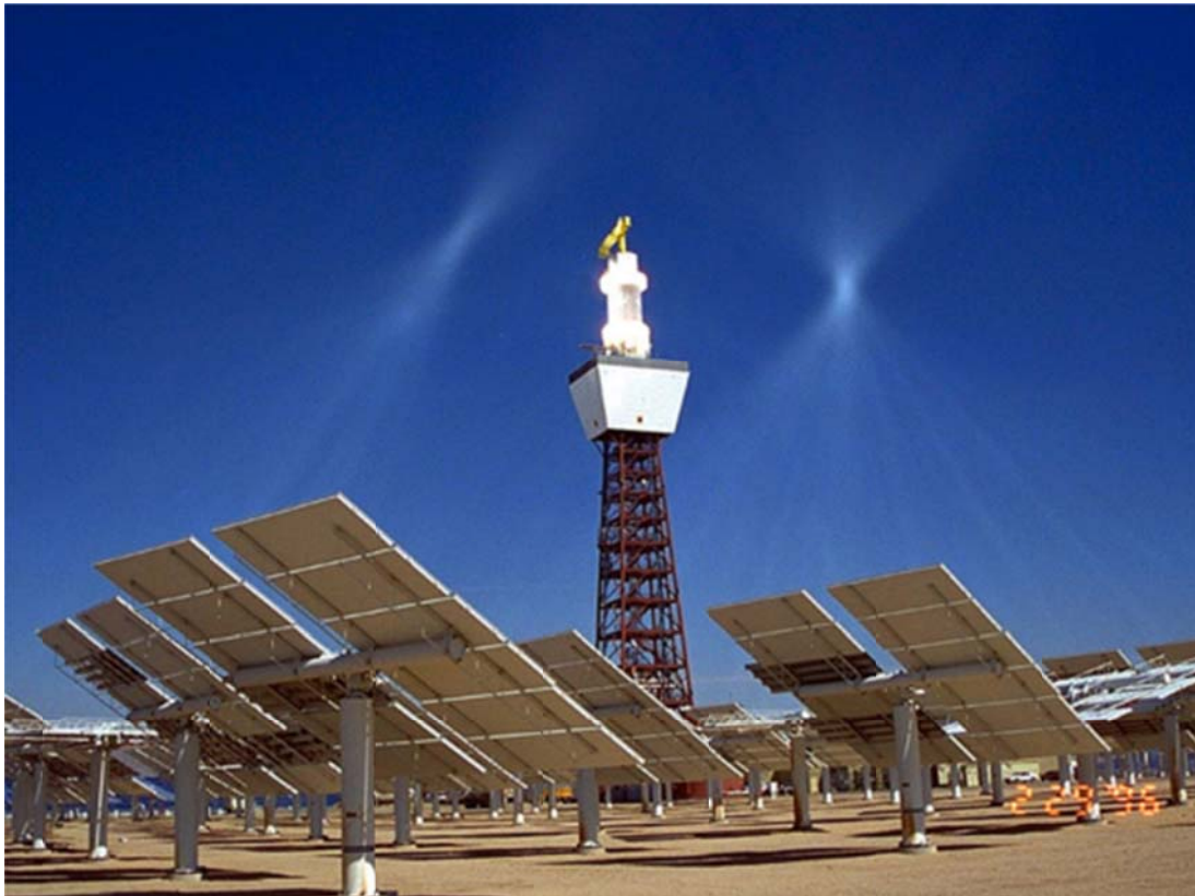
Photo 2. Solar One Standby Points which caused bird burn mortality.
