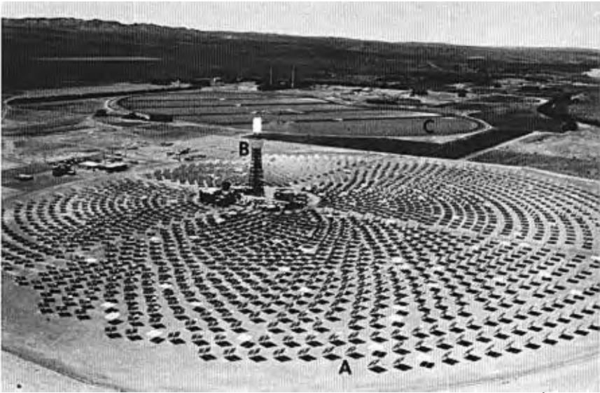
FIGURE 1. Aerial view of Solar One: (A) heliostat field, (B) central receiver tower, (C) evaporation ponds. Tower height = 86 m, diameter of field = 765 m.
