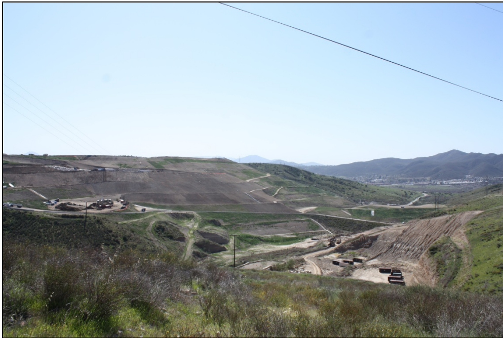
Figure 5-24. Overview of Sycamore Landfill (South)
