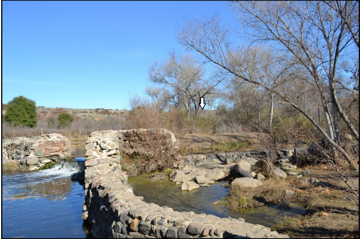
Figure 4-3. Photograph of Mission Dam Looking Northeast Toward APE, January 2012
