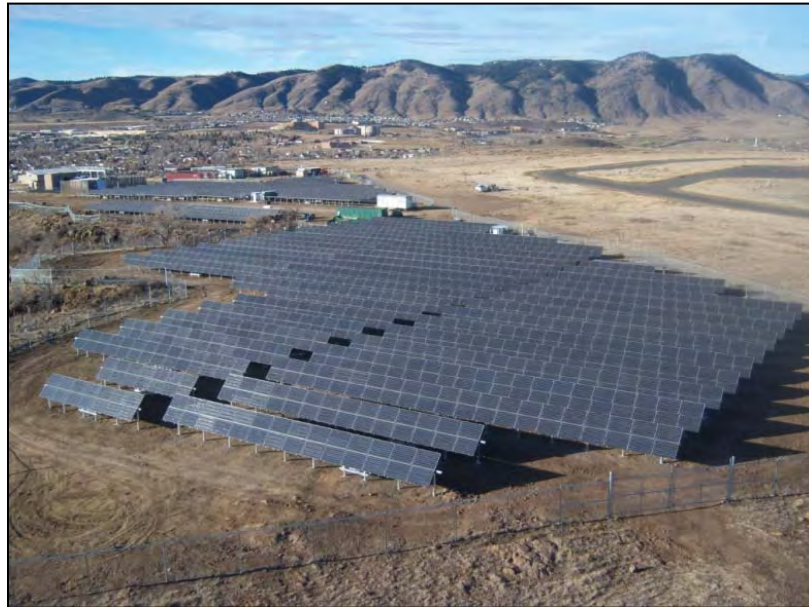
Figure 73. 720 kW Single axis tracking system at NREL (Credit: Patrick Corkery, NREL)
