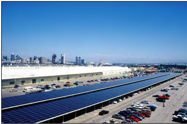
Figure 70. Carport PV at Coronado Island, CA (Courtesy of SunPower)
