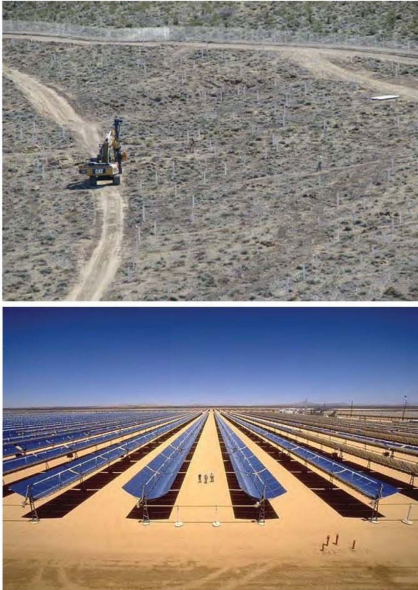
Figure DR 86-1. Minimal ground disturbance of power tower technology solar field relative to parabolic trough solar field
