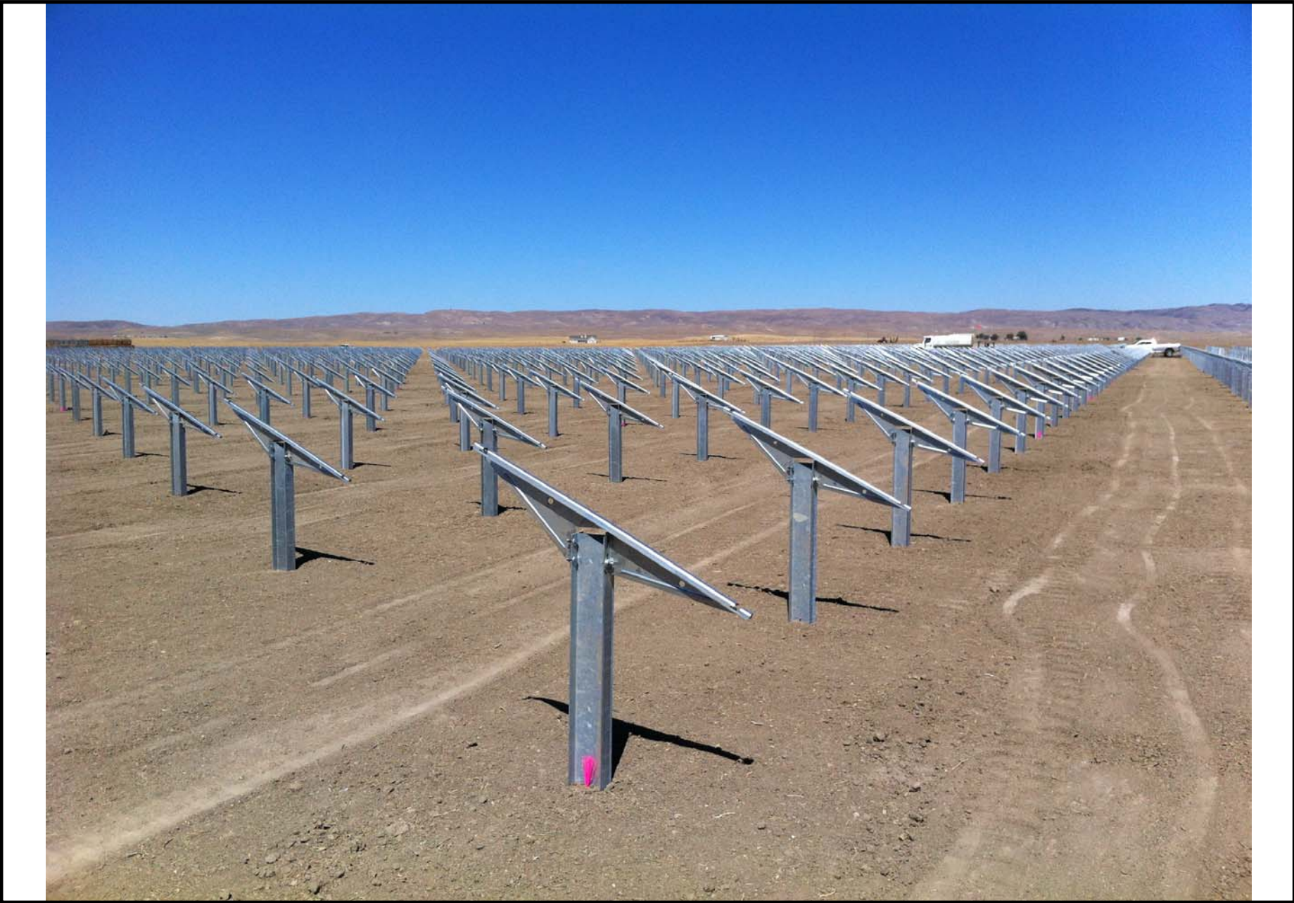
Hidden Hills Solar Electric Generating System (HHSEGS) - Site Preparation and Revegetation at the Topaz Solar Farm Project Site - PV Array Block 6 after Installation of Posts and Tilts
