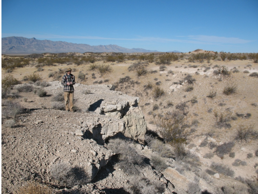
Photo DR105-4. A lithoid tufa ledge exposed on the north side of an arroyo in the SFS. It caps and protects less resistant bedded silts and clays below it. To the right of the man, across the arroyo, the linear white area reveals an exposure of the tufa ledge on the other bank, largely obscured by a sand sheet that mantles the downwind wall of the arroyo. View northwest. Note the coppice dunes in the background.
