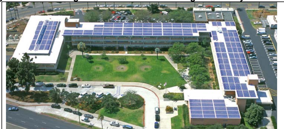
Figure 10-3. San Diego Education Center with High Efficiency Roof and PV
