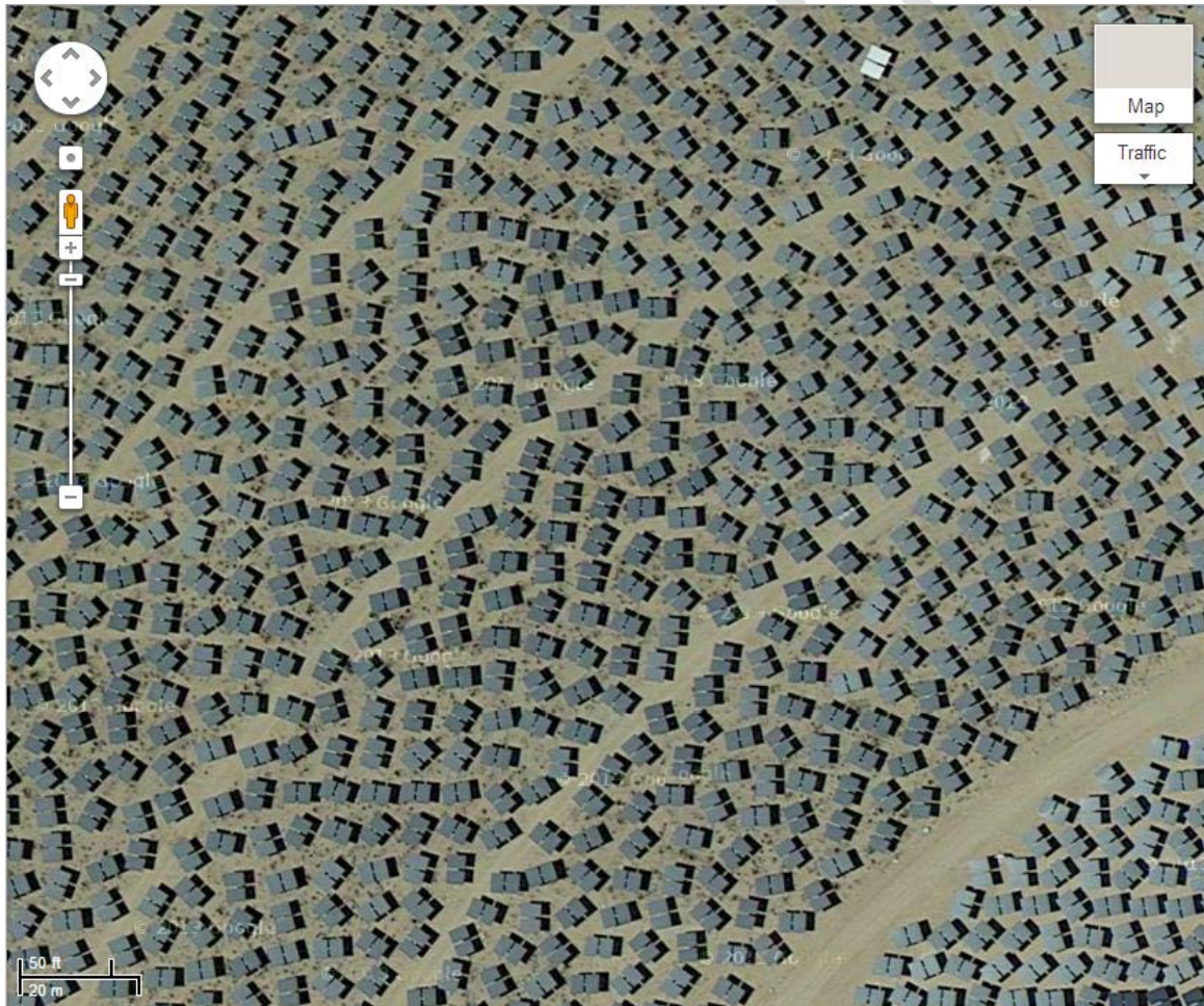
Figure 6: The Ivanpah Solar Electric Generating System as seen via satellite. The mirrored panels are 5 x 8 feet.
