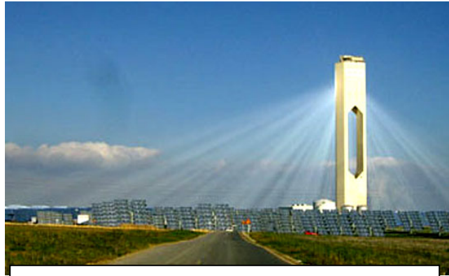
Figure 8: Seville solar power facility ( http://inhabitat.com/sevilles-solar-power-tower )
