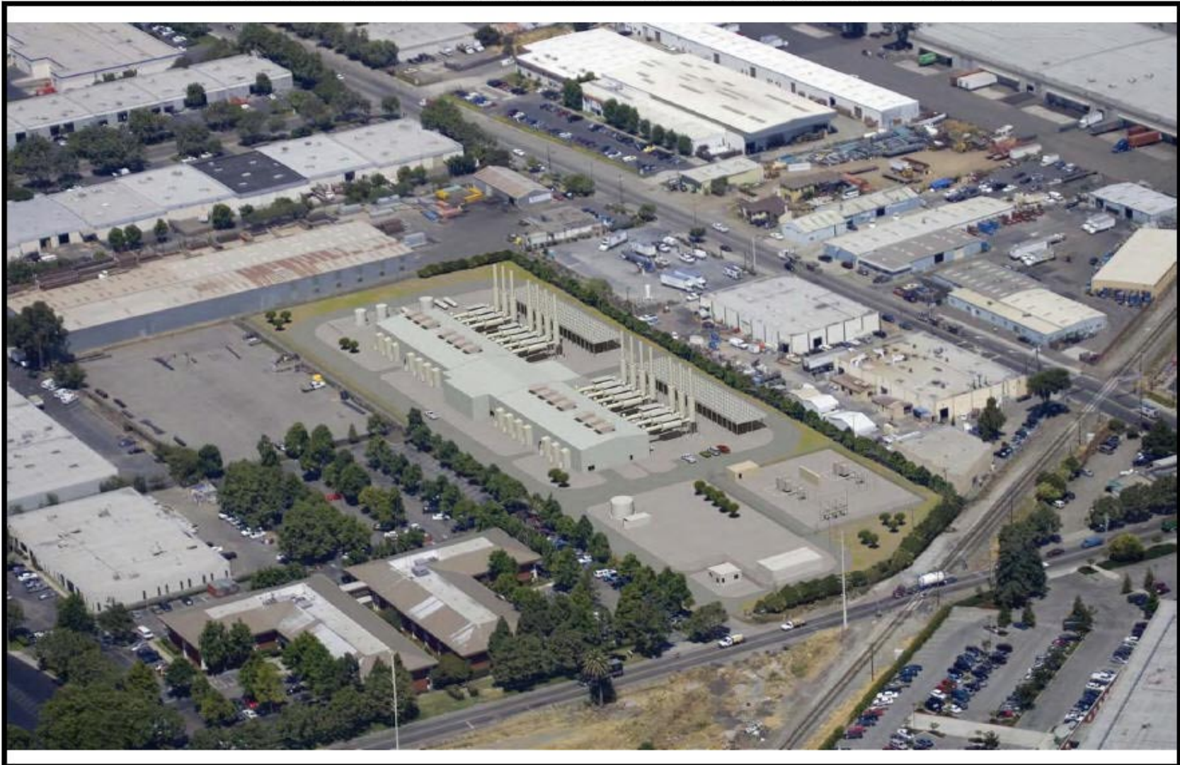
Eastshore Energy Center - Bird's Eye View of a Photo Simulation of the Proposed Project After Completion
