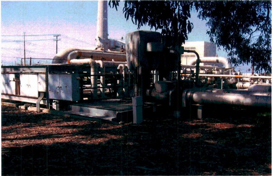
Photo 21: View of the fuel oil re-load/un-load pumps.
