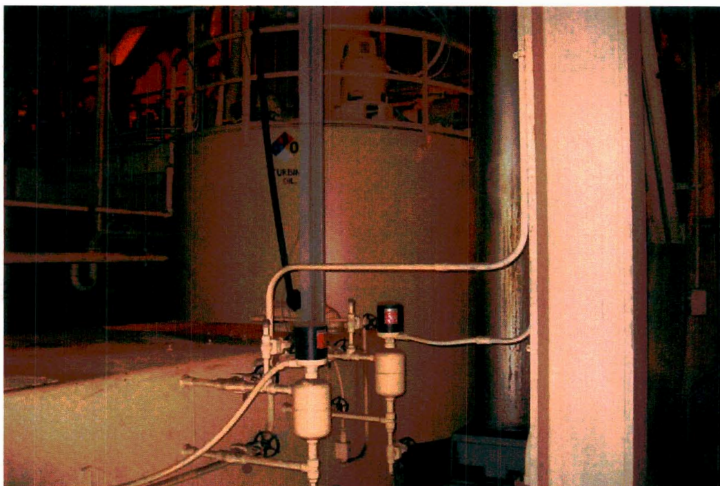
Photo 6: View of typical AST located inside the Encina Power Station used to store turbine oil.
