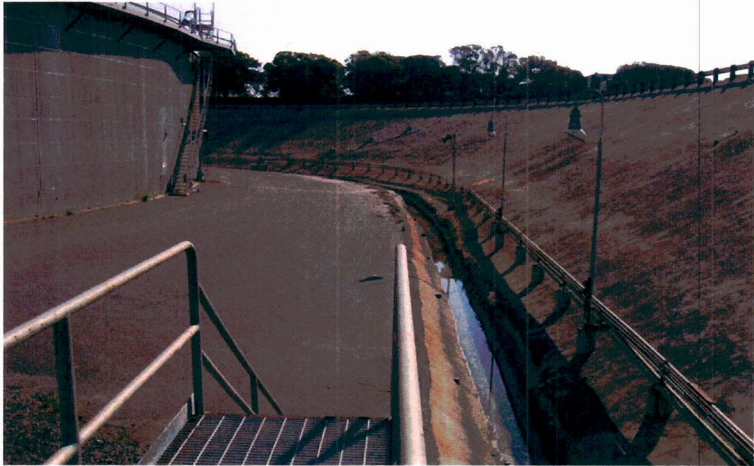
Photo 29: View of typical secondary containment system for AST Nos. 4, 5, 6, and 7.
