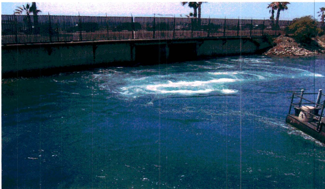
Photo 37: View of the discharge basin for the Encina Power Station. Discharge water flows under Carlsbad Boulevard (shown) to the Ocean (not visible).
