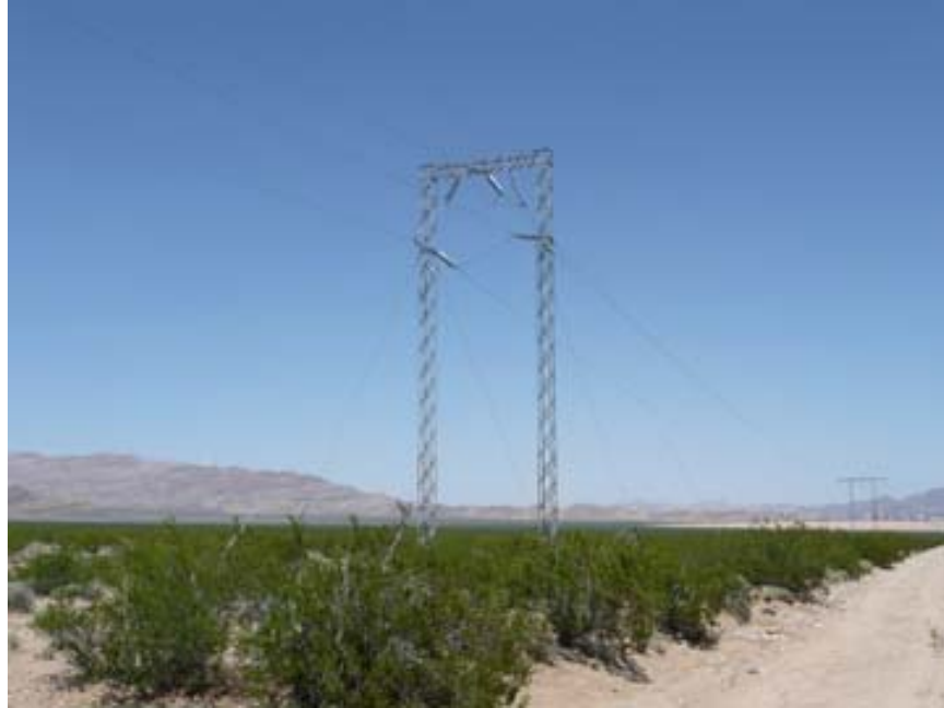
Photograph 3. Original transposition tower, camera facing north, December 10, 2007.
