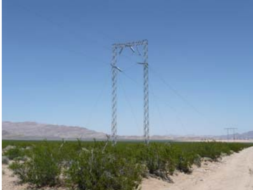
Photograph 3. Original transposition tower, camera facing north, December 10, 2007.
