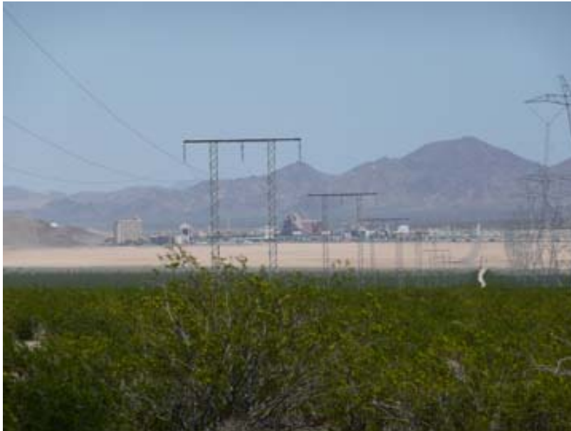
Photograph 1. Showing 1931 Boulder Dam-San Bernardino 138 kV transmission line on left with the newer Los Angeles Metropolitan Water District 500 kV transmission line on the right, City of Primm in background with Interstate Highway 5, camera facing northwest, December 10, 2007.
