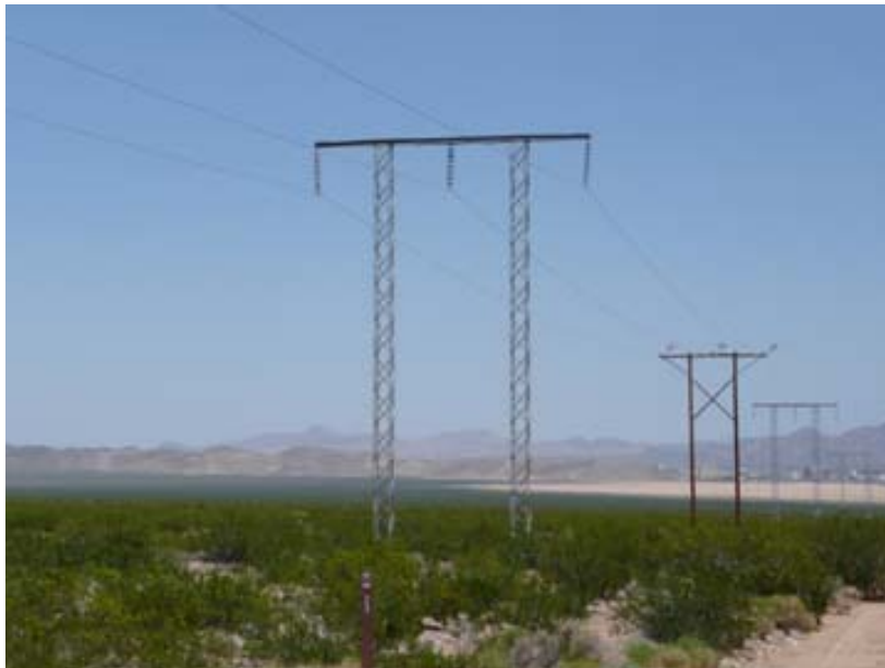
Photograph 2. Showing original tower in foreground and replacement wood tower in background, camera facing northwest, December 10, 2007.
