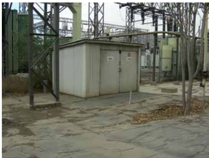
Photograph 13. Service Shed 1, camera facing northwest.
