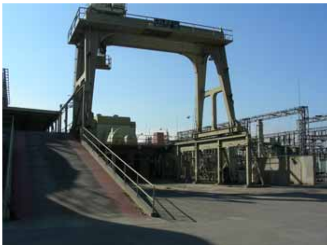
Photograph 9. Traveling service crane, camera facing southwest
