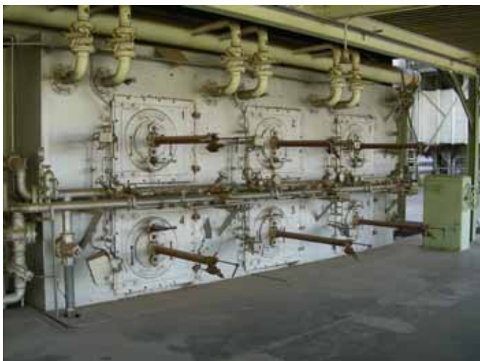
Photograph 5. Unit 1 boiler doors, camera facing southeast
