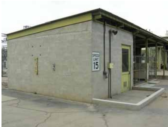
Photograph 15. Hazardous Materials Building, camera facing northwest.
