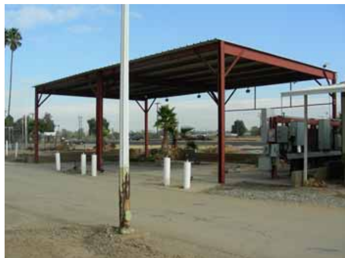
Photograph 23. Vehicle shelter, camera facing northeast.
