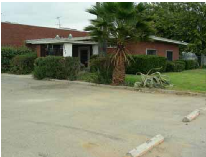
Photograph 2. Administration Building, camera facing northwest
