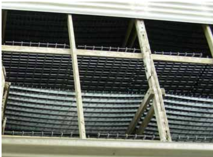
Photograph 18. Interior of Cooling Tower 3 showing metal gridwork. Camera facing north.
