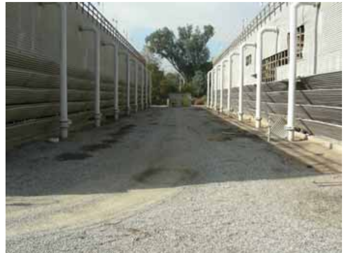
Photograph 17. Pipes entering Cooling Towers 1 and 2, camera facing west.
