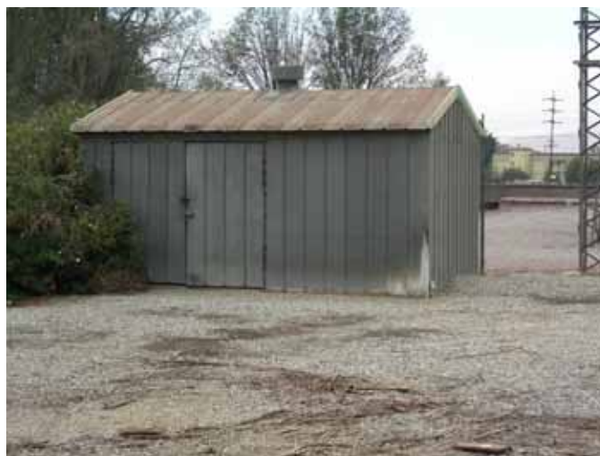
Photograph 14. Service Shed 2, camera facing southwest.
