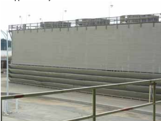
Photograph 16. Cooling Tower 1, camera facing southeast.
