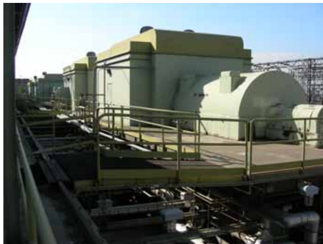
Photograph 10. Generator deck, camera facing southwest
