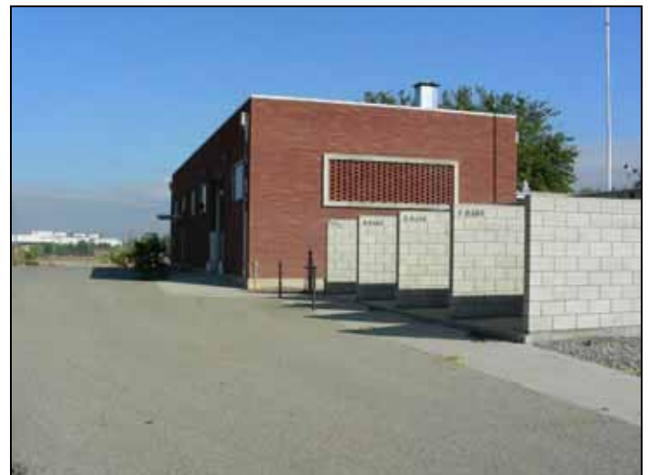
Photograph 3. Administration Building, camera facing north
