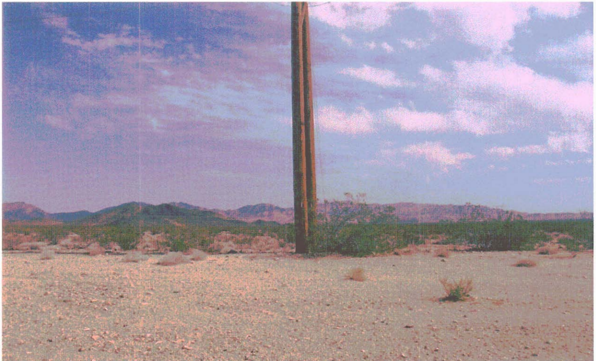
Figure 2: Picture of the Subject Property taken from Yates Well Road, facing north
