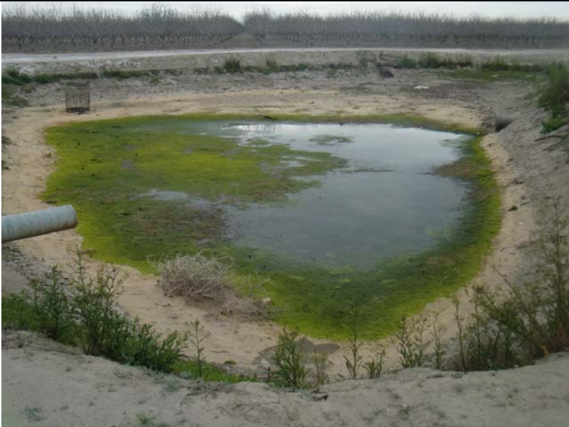
Photograph 10 – View of a typical retention/detention basin in study area (NJ 33).
