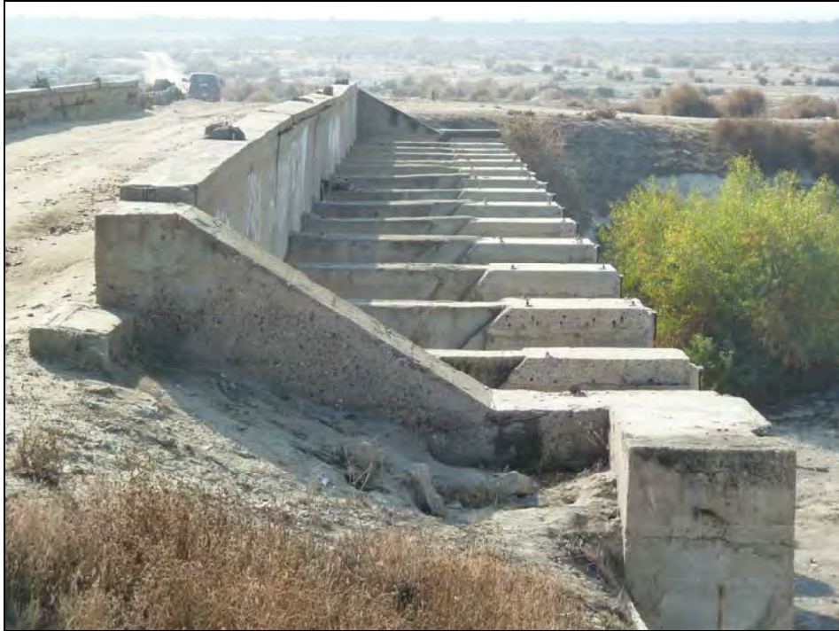
Photograph 2: East side of Weir, showing location of former walkways, camera facing south.
