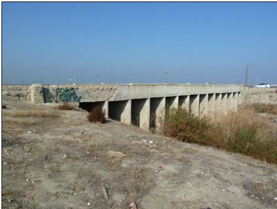
Photograph 6: East side of weir, camera facing northwest.
