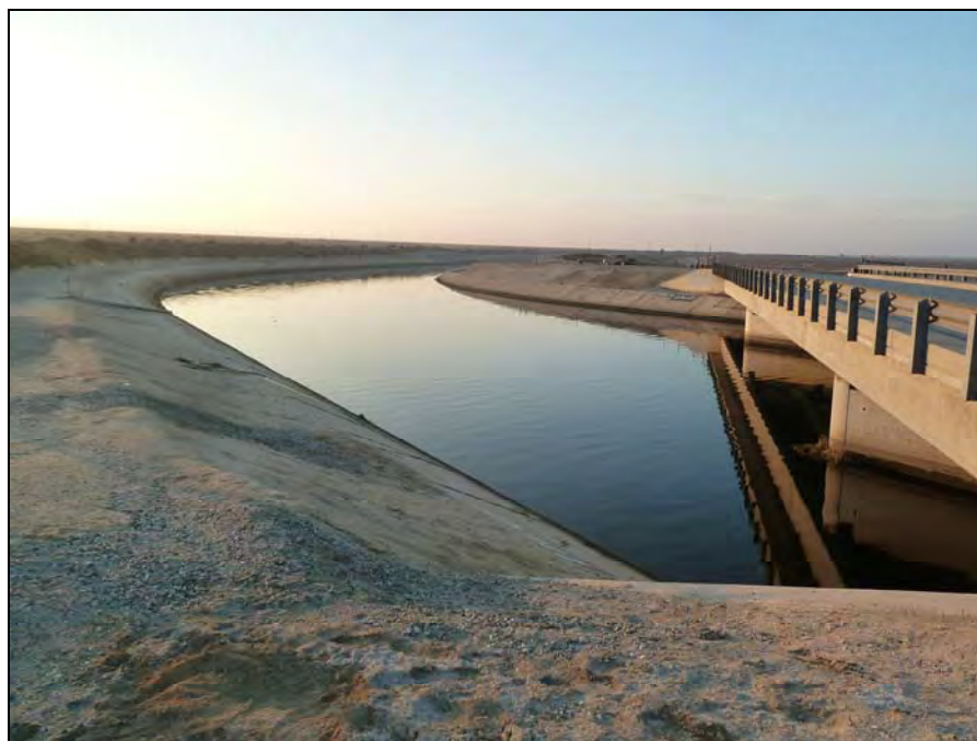
Photograph 1: View of the California Aqueduct at Tupman Road (see Point 1 on sketch map), camera facing west.
