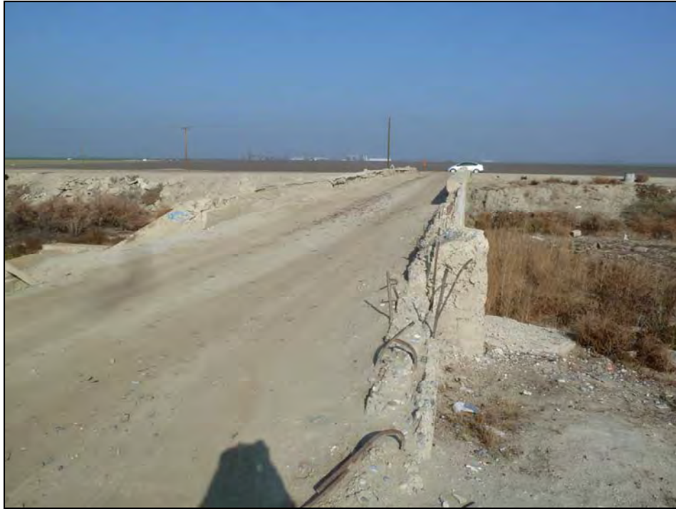
Photograph 8: Deck/top of weir, camera facing north.
