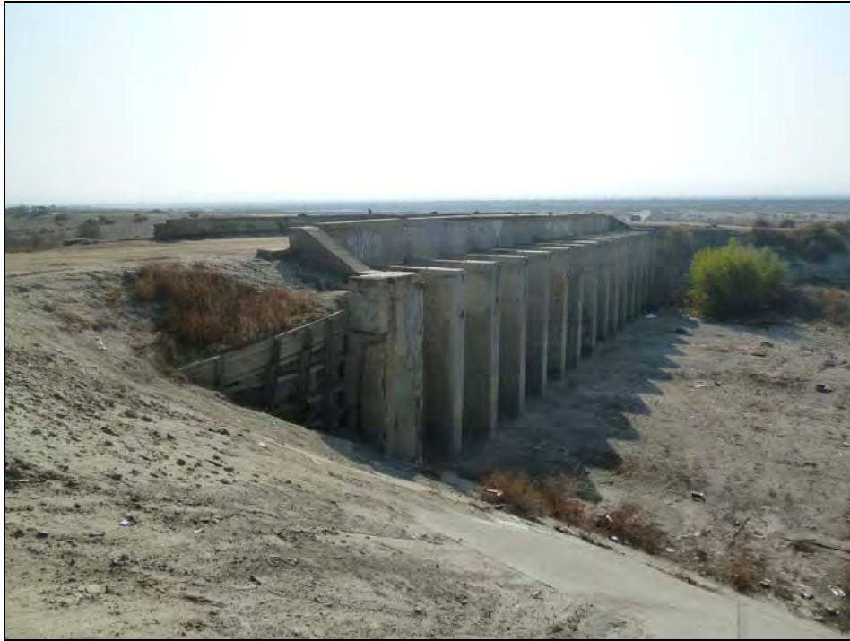
Photograph 4: West side of weir, camera facing south.
