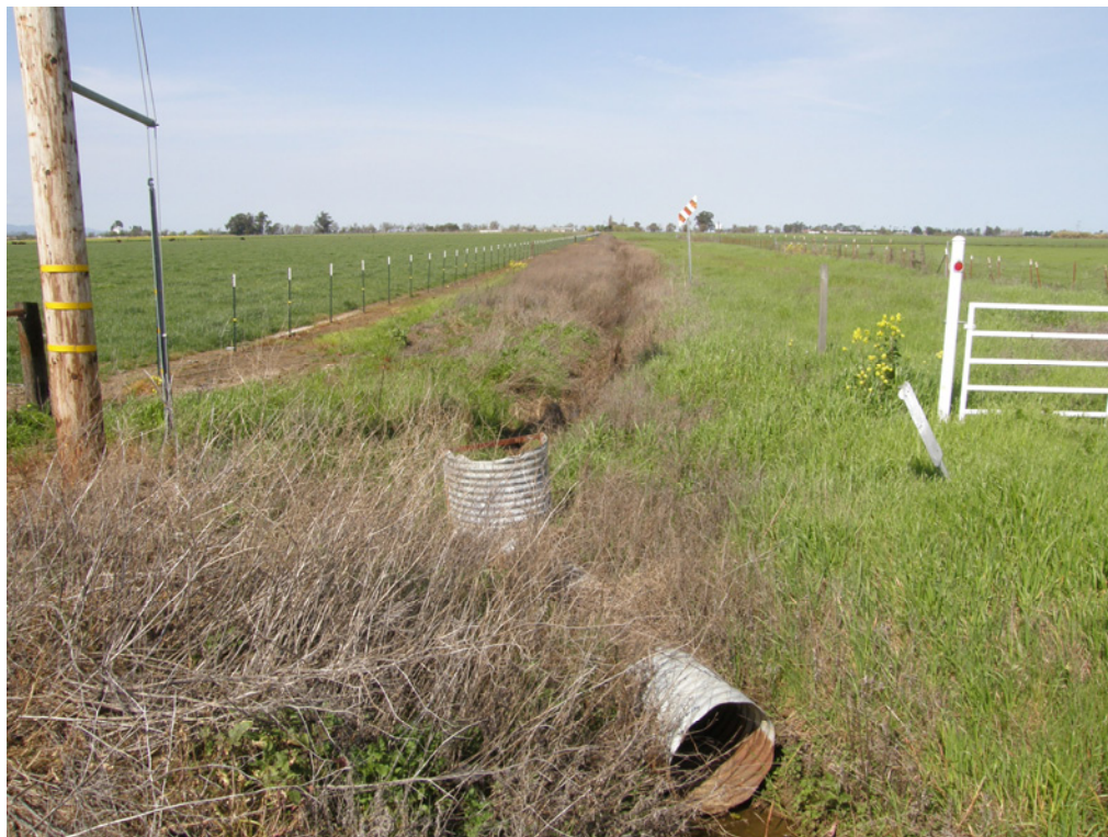
PHOTO 24 AD-14, to the North. (March 17, 2009)
