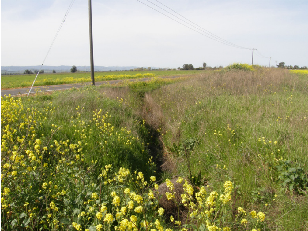
PHOTO 11 AD-03P Culvert Inlet, to the Southwest. (March 17, 2009)
