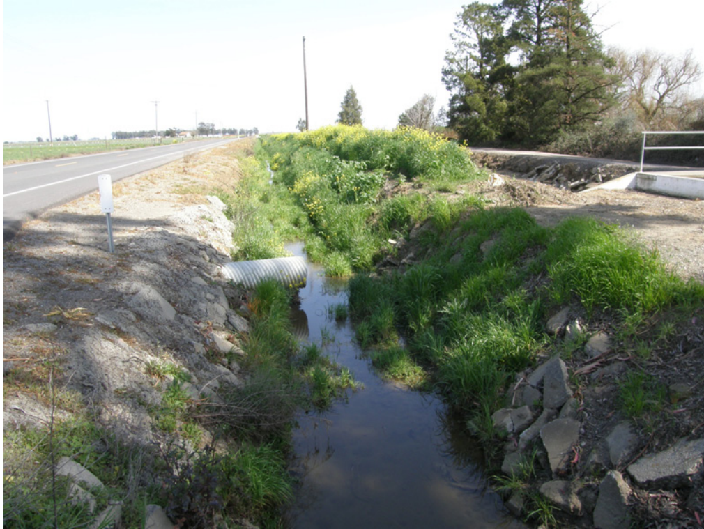
PHOTO 23 AD-11 Showing Outfall to Eastern Primary Drainage, to the East (March 17, 2009)
