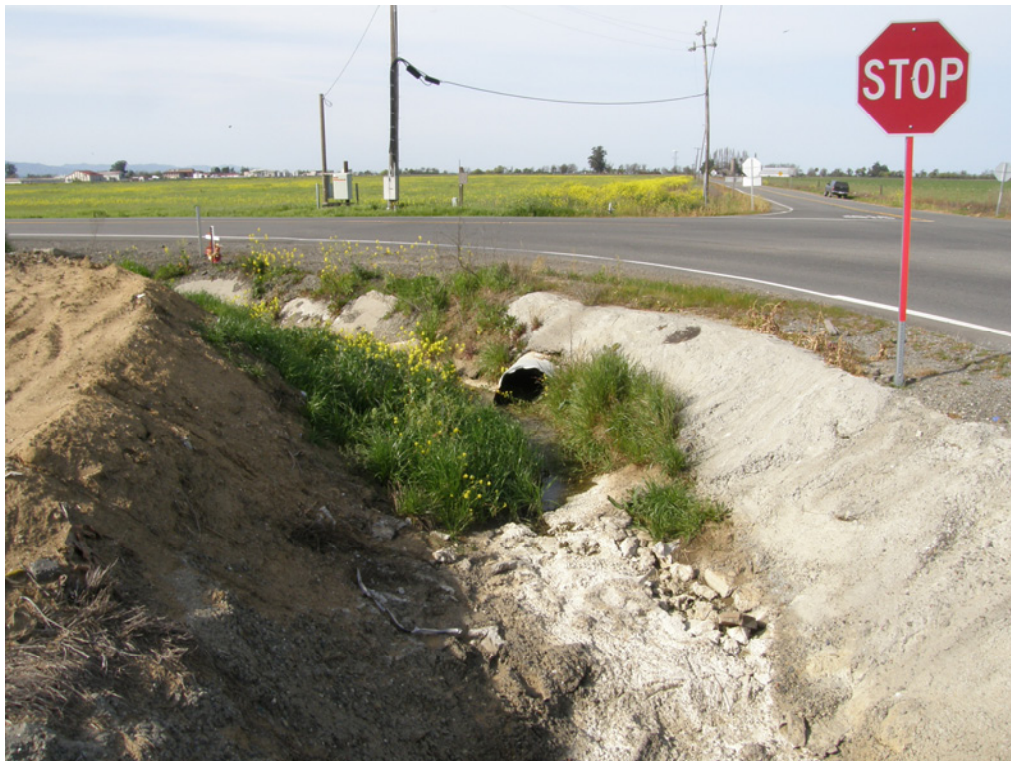
PHOTO 14 RD-06 Outfall to the Western Primary Drainage, to the North. (March 17, 2009)
