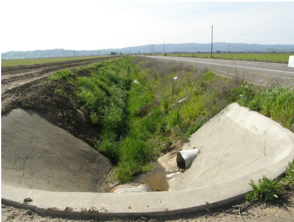
PHOTO 12 RD-05 Outfall to the Western Primary Drainage, to the West. (March 17, 2009)
