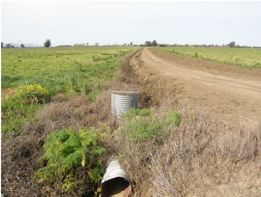
PHOTO 6 AD-02, to the North. (March 17, 2009)
