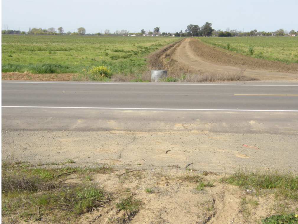
PHOTO 7 AD-02, Showing Unpaved Access Road above Culvert to Western Primary Drainage, to the North. (March 17, 2009)
