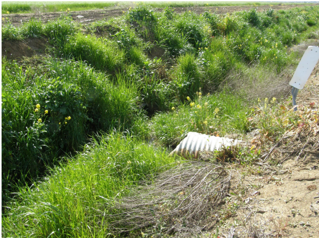
PHOTO 18 AD-08 Outfall to the Eastern Primary Drainage, to the Southwest. (March 17, 2009)
