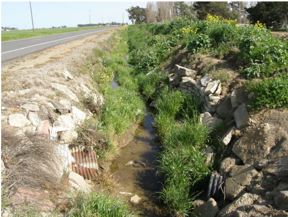
PHOTO 20 AD-09 Outfall to the Eastern Primary Drainage, to the East. (March 17, 2009)
