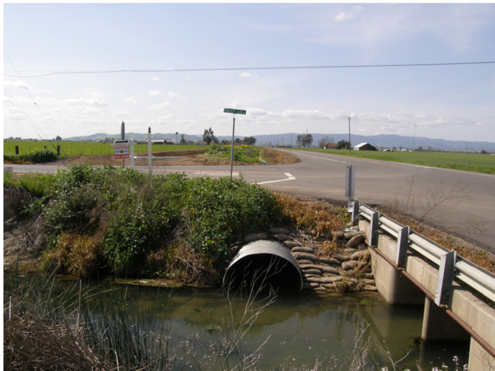
PHOTO 2 Confluence of Eastern Primary Drainage with Old Alamo Creek, to the West. (March 17, 2009)
