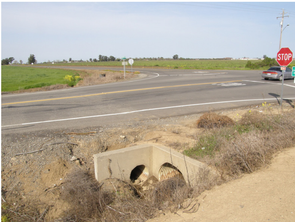
PHOTO 4 RD-01 Outfall to the Western Primary Drainage, to the Northeast. (March 17, 2009)
