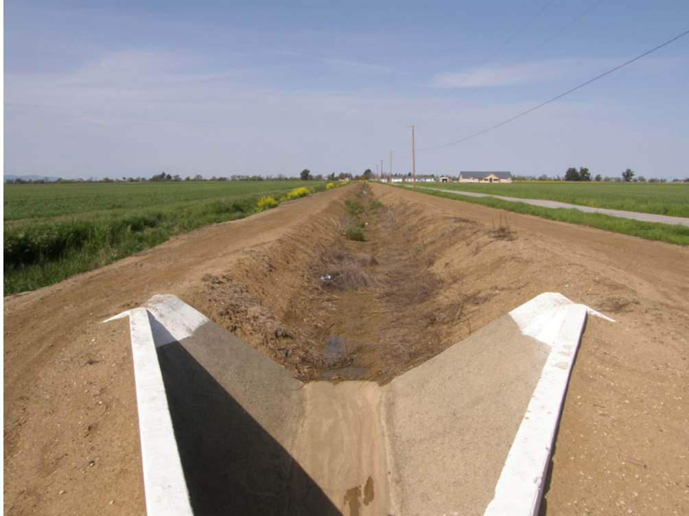
PHOTO 21 AD-10, to the North. (March 17, 2009)
