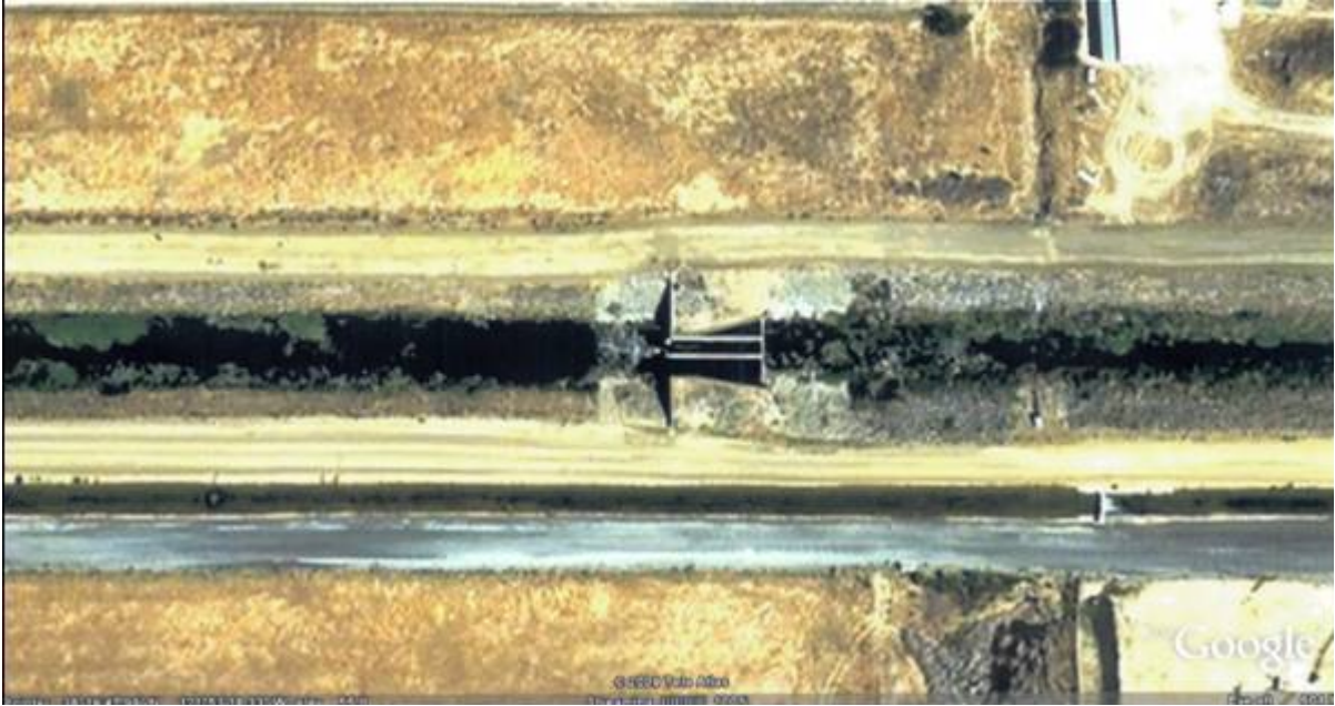
FIGURE 4-1 Aerial View of Grade Control Structure at New Alamo Creek Acting as Barrier to Fish Passage at RM 4.2
