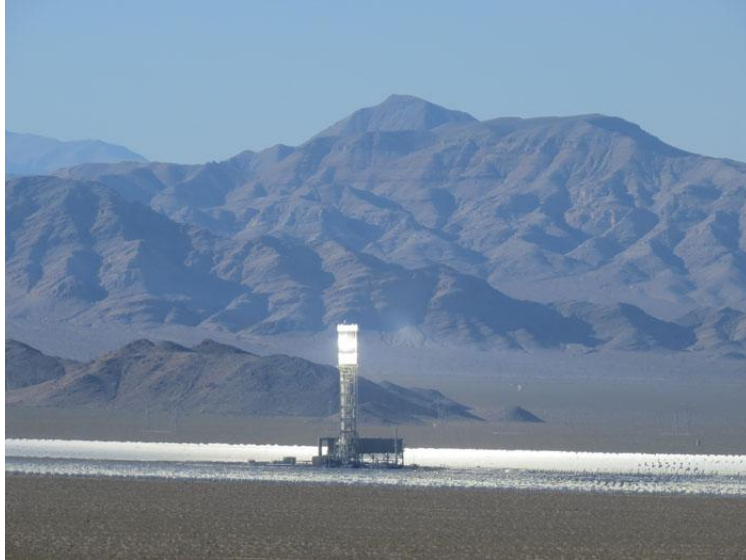
^Ivanpah Solar Electric Generating System, June 2013
