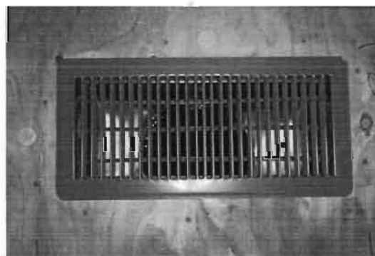
Figure 5 Example supply grille of multi-branch duct system.
