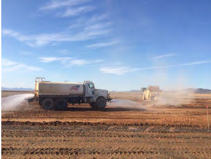
Photo 5: AQ SC-3: Construction Fugitive Dust Control Dust abatement on Unit 1 ripping and grading; August 10, 2015
