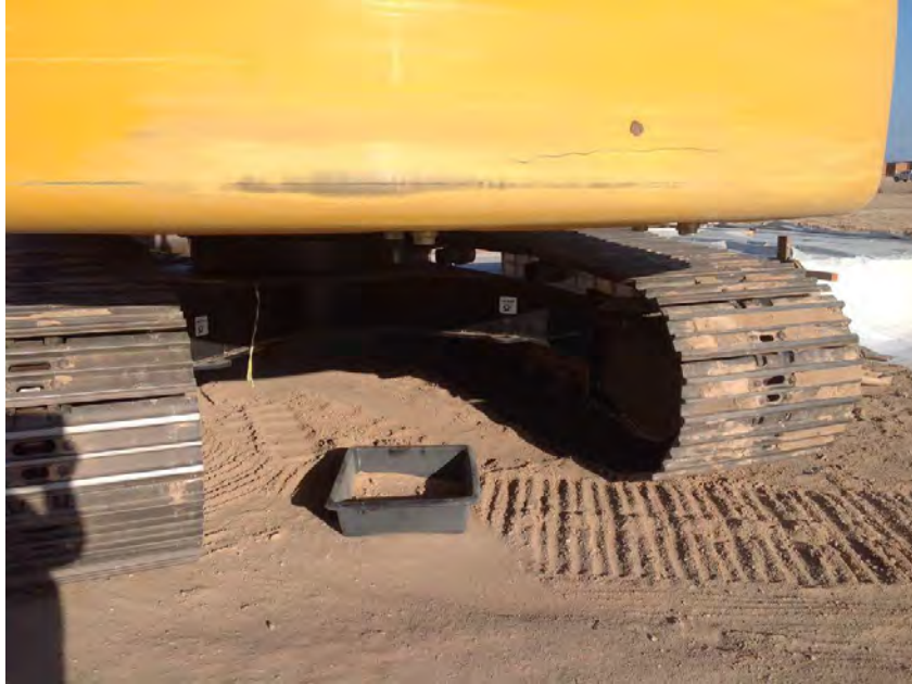
Photo 9: DF Bio-8: Minimize Spills of Hazardous Materials Drip pan used underneath excavator in Unit 1; August 22, 2015
