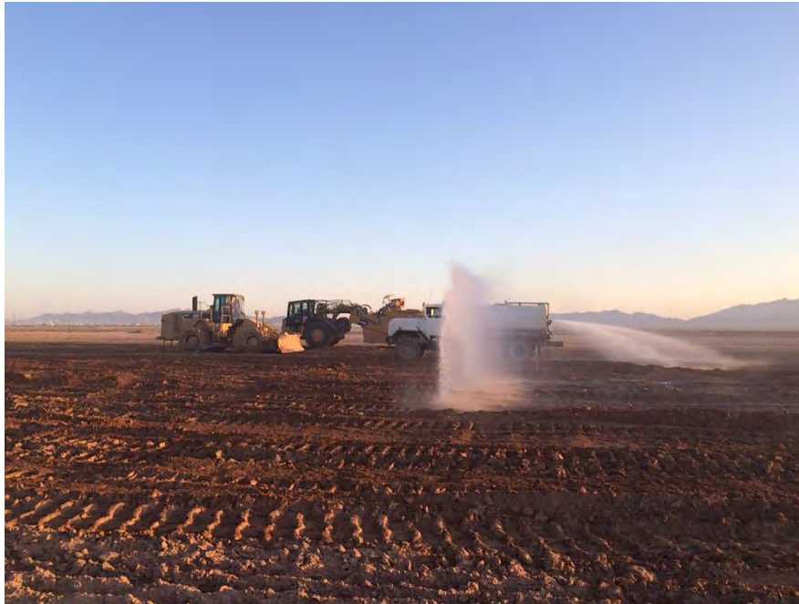
Photo 10: AQ SC-3: Construction Fugitive Dust Control Dust abatement on Unit 1; August 24, 2015
