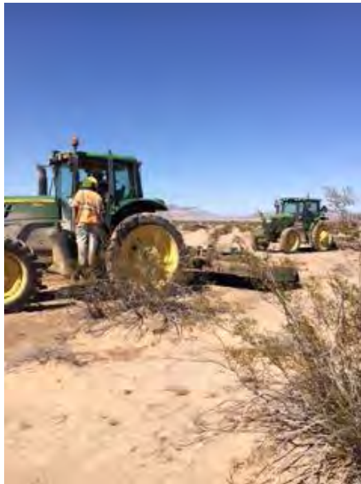
Photo 2: DF Bio-8: Monitor During Construction
