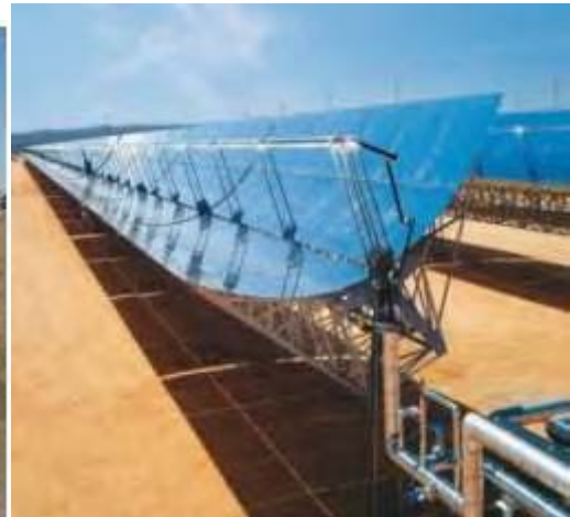
Completed Solar Trough Assembly
