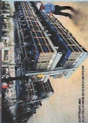
100 kW, 15 kWh lithium battery for UPS applications
