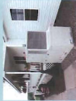
100 kW, 15 kWh lithium battery for UPS applications
