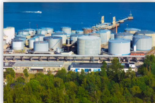
Fuel storage facility in Stockholm, Sweden.
