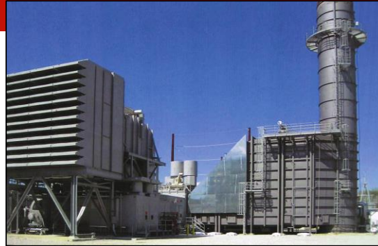
LMS100 Gas Turbine Generator with size 272T SSS® Encased Clutch at Calpine (formerly Conectiv) Cumberland Energy Center, Millville, NJ.
