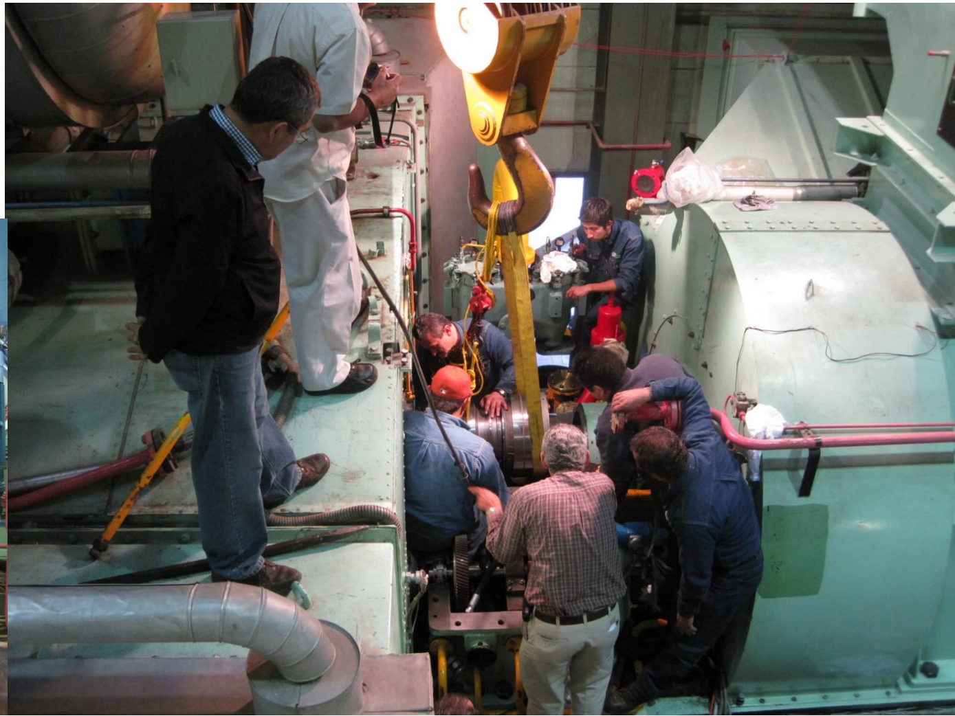
Installation of size 160FT SSS Clutch into BB11-L
