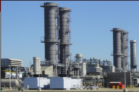
Two LMS100 Gas Turbine Generators with size 272T SSS® Encased Clutches at LADWP's Haynes Power Station, Long Beach, CA
