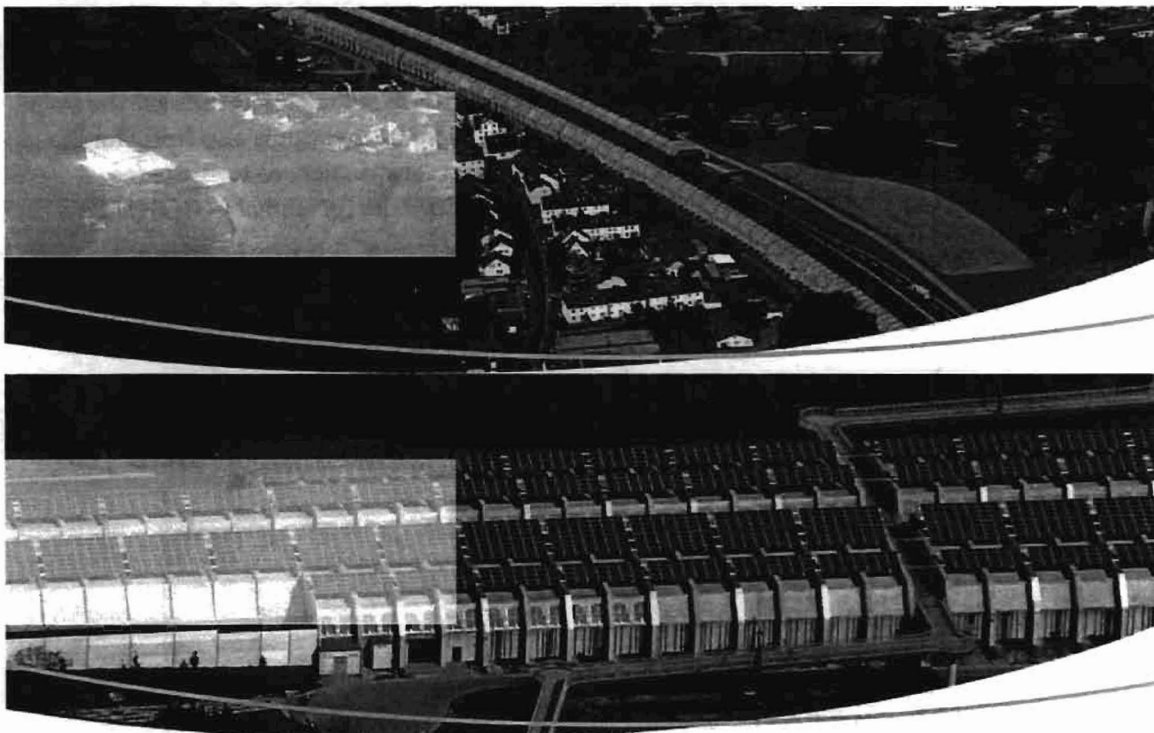
Figure 3: A Pioneer 1.6 MW Project for Enclosure of Transportation Noise on Highway A3 between Goldbach and Hösbach. 12
