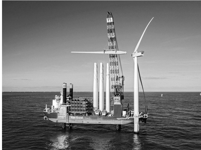
Gemini offshore wind farm, under construction
