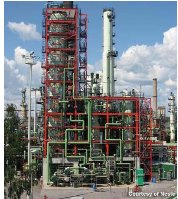
NExBTL-diesel started at the Porvoo refinery in 2007.
