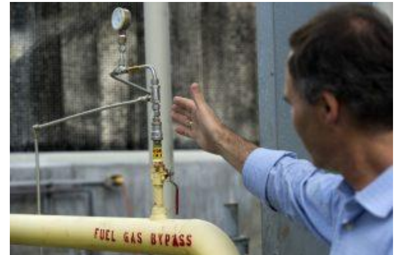
Hydrogen Injection into UCI NGCC Power Plant
