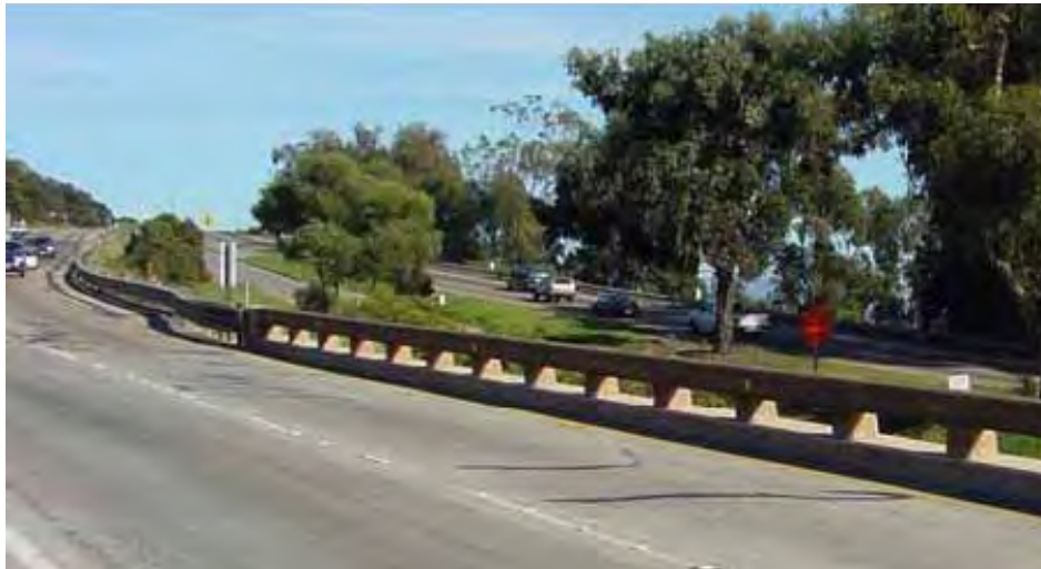
Figure 3-7.144: Type 80 bridge rail
