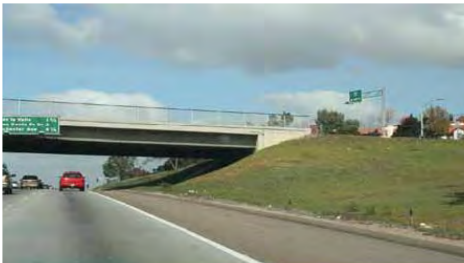
Figure 3-7.136: An example of a short seat abutment
