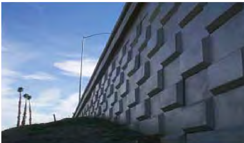
Figure 3-7.135: An MSE wall with a four-in pattern reveal
