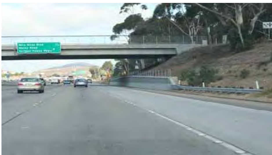
Figure 3-7.137: Secondary walls such as this reduce visual unity and should be avoided
