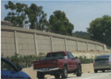
The Lomas Santa Fe interchange retaining walls in Salinas Beach.
