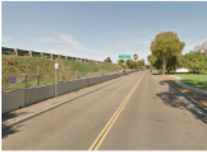
The view from Pio Pico in Cochise where a viaduct wall would be used
