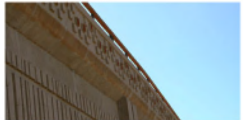
Example of Selma Beach wall
