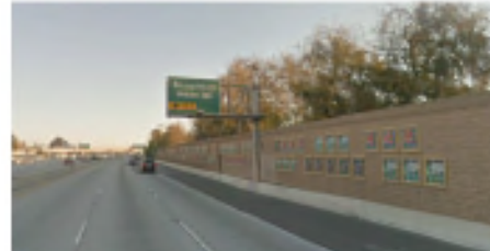
Interchange detail is not perceived by the freeway traveler along I-15 in this example in Orange County
