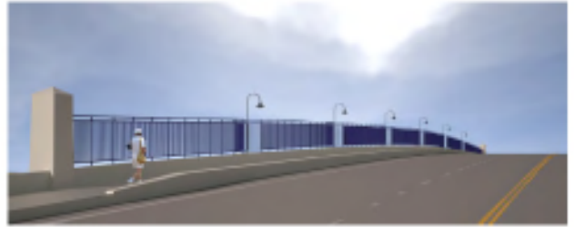
Perspective from bridge approach
