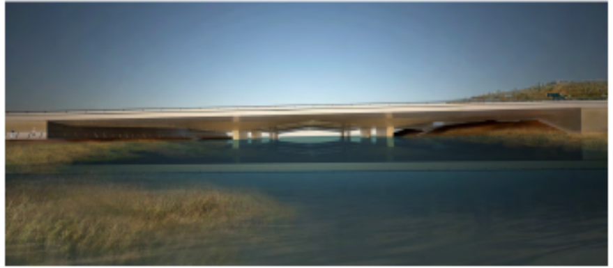
Elevation view of the lagoon bridge.
