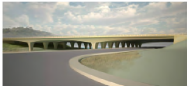
View of lagoon bridge looking southwest
