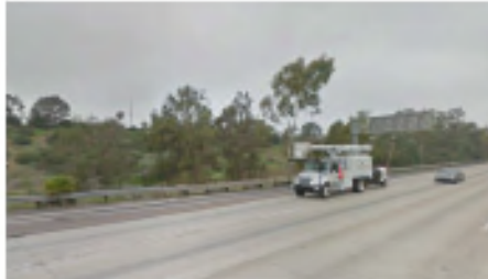
Cottonwood Creek adjacent to the freeway in Encinitas
