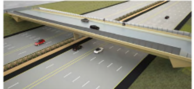
Aerial view of overcrossing
