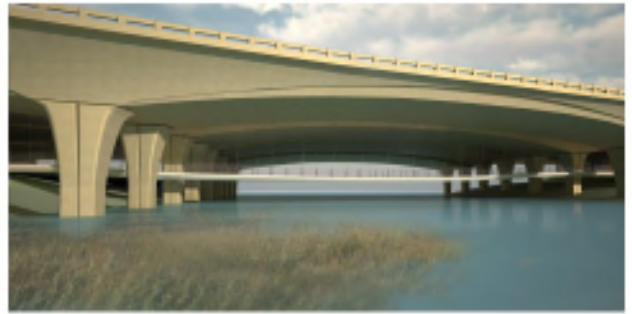
Pedestrian bridge suspended from main structure
