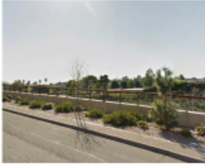
Alternative access control barrier in Delana Beach
