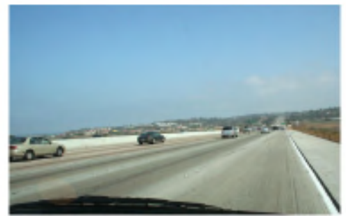
The horizontal is emphasized next to the freeway creating a need for vertical elements
