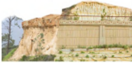
In Solana Beach, the natural character of the surrounding bluffs was the basis for the design of the walls.
