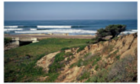
Encina Creek Bridge
