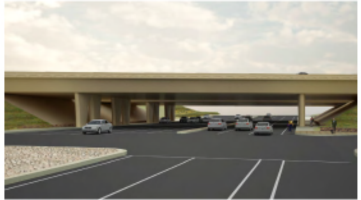
View of gateway from approach with columns at front of sidewalk
