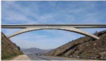
The West Line Road Bridge over Interstate 15
